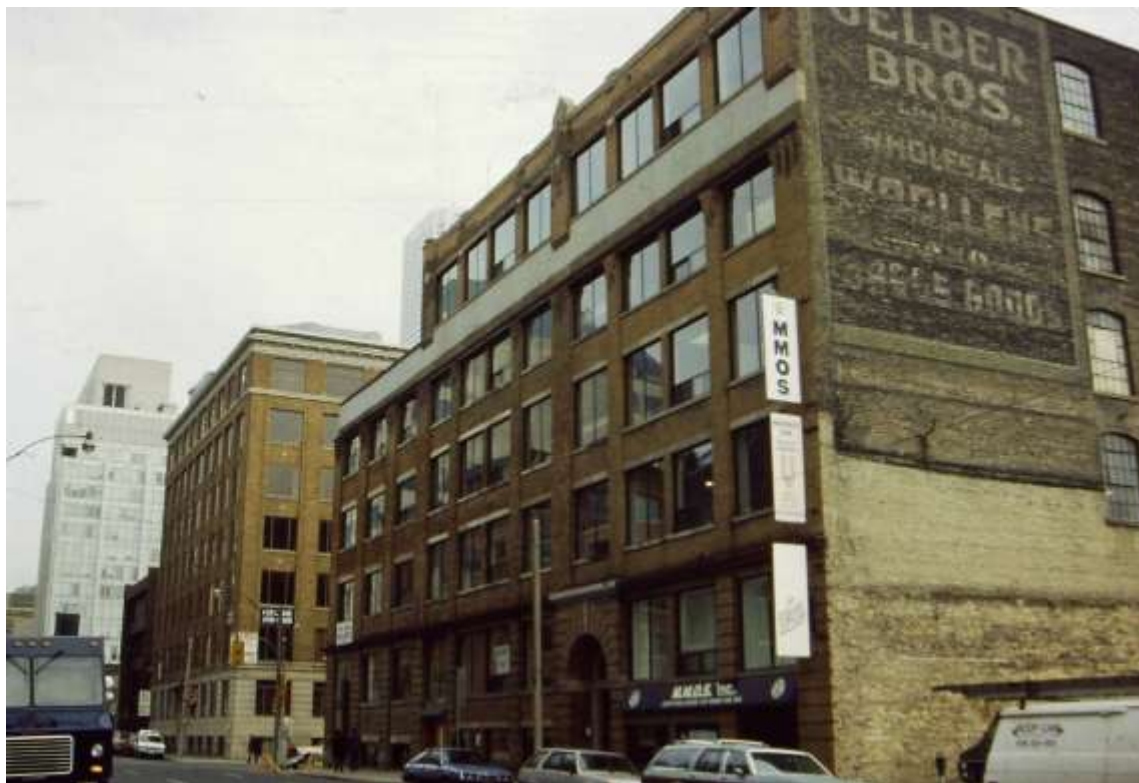
10. Richmond Street looking west with the Gelber Building on the right showing the "Gelber Brothers Limited" signage on the west façade, the five-and-a-half storey addition designed by Brown in 1923 and the original, four-and-a-half storey Gelber Building designed by Louis S Yolles in 1910 to the left. Across Duncan Street, to the left, is the New Textile Building, commissioned by the Gelbers in 1923-4 and designed by Brown. (Toronto Historical Board, April 1991)
