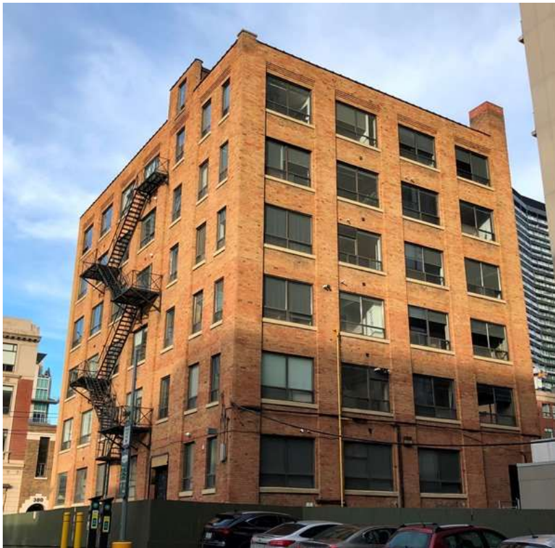
34. Side (west) and rear (south) facades of the building at 355-359 Adelaide Street West (HP, 2020)
