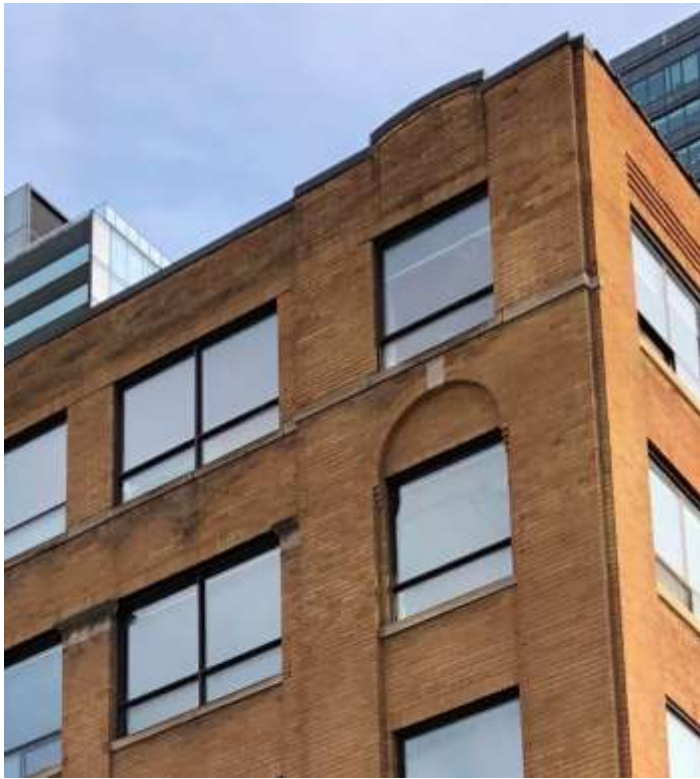
32. Photograph showing the details at the upper stories of the principal (north) elevation including the stone sills and belt courses, the stone caps on the pilasters, the arch with keystone and the stepped brick supporting the arch, the panel with its curved head raised above the parapet and the stepping forward of the outer bay. Note also on the side elevation, the stepped bricks above the top floor window (HP, 2020)
