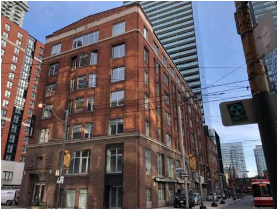
36. MacLean Building, 1914, 345 Adelaide Street West at the intersection with Charlotte Street to the east of 355-359 Adelaide Street West. The building represents a similar typology in terms of scale, design and details. (HP, 2020)
