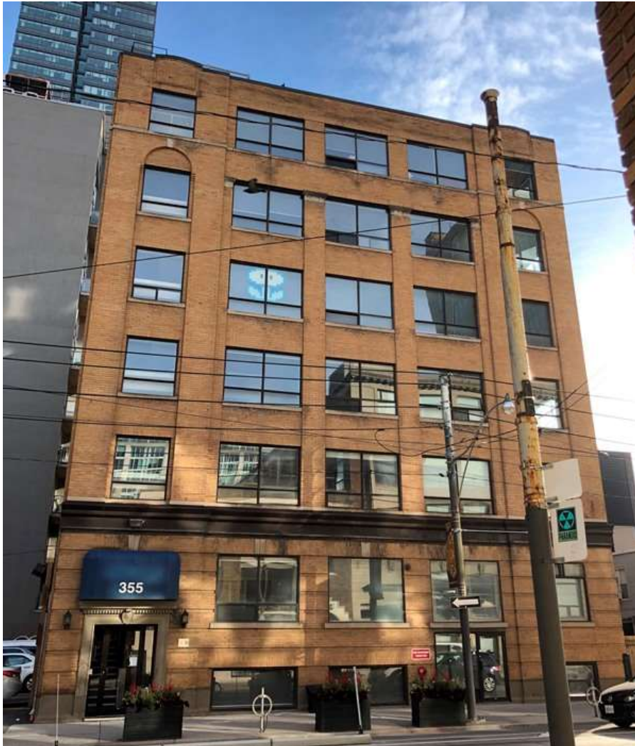
355-359 Adelaide Street West, principal (north) facade (Heritage Planning, 2020)
