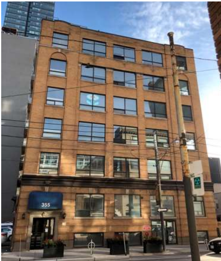
29. 355-35 Adelaide Street West, Principal (north) elevation (HP, 2020)
