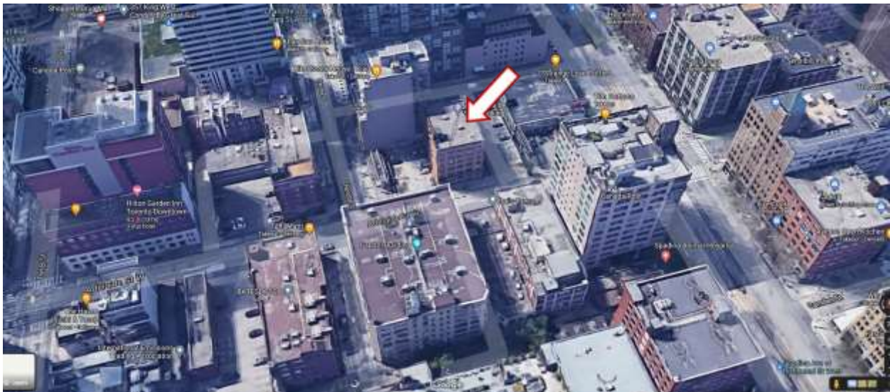
2. Aerial view of the property at 355-359 Adelaide Street West, looking south. (Google Maps, 2020)
