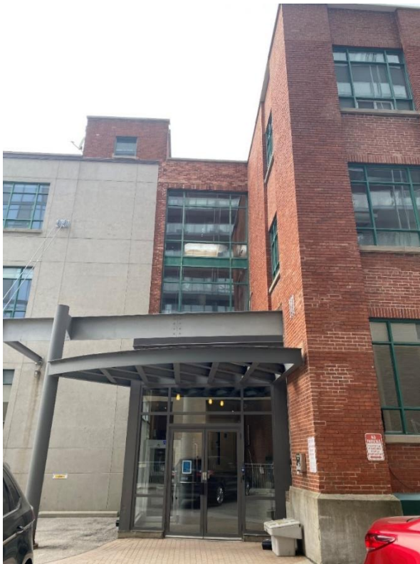
Figure 10: Current photo looking north and showing the later entrance and steel canopy by Moriyama & Teshima Architects added to the Frankel Building where the 1915 and 1925 buildings connect. The firm also installed the horizontal brise-soleil over the first-floor windows on the principal (west) elevation. (Heritage Planning, 2021)
