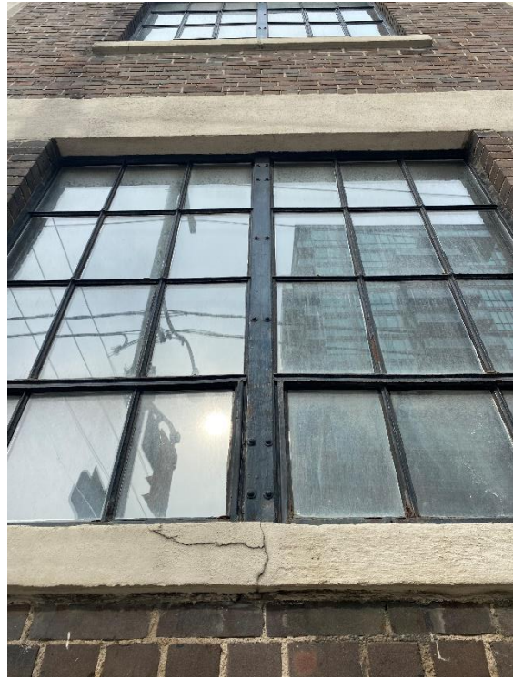
Figures 21 and 22: Current photos of 125 George Street showing the Georgian style main entrance constructed of precast concrete (left) and the steel framed and mullioned industrial windows found on all elevations except the blind south wall. (Heritage Planning, 2021)
