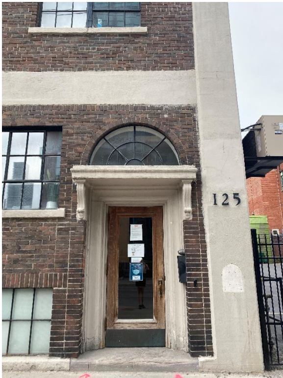
Figures 21 and 22: Current photos of 125 George Street showing the Georgian style main entrance constructed of precast concrete (left) and the steel framed and mullioned industrial windows found on all elevations except the blind south wall. (Heritage Planning, 2021)
