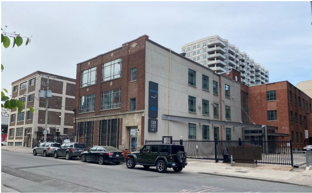
Figure 15: Current contextual photo looking northeast and showing both subject properties as well as the stucco overcladding on the south elevation at 109-117 George Street. (Heritage Planning, 2021)
