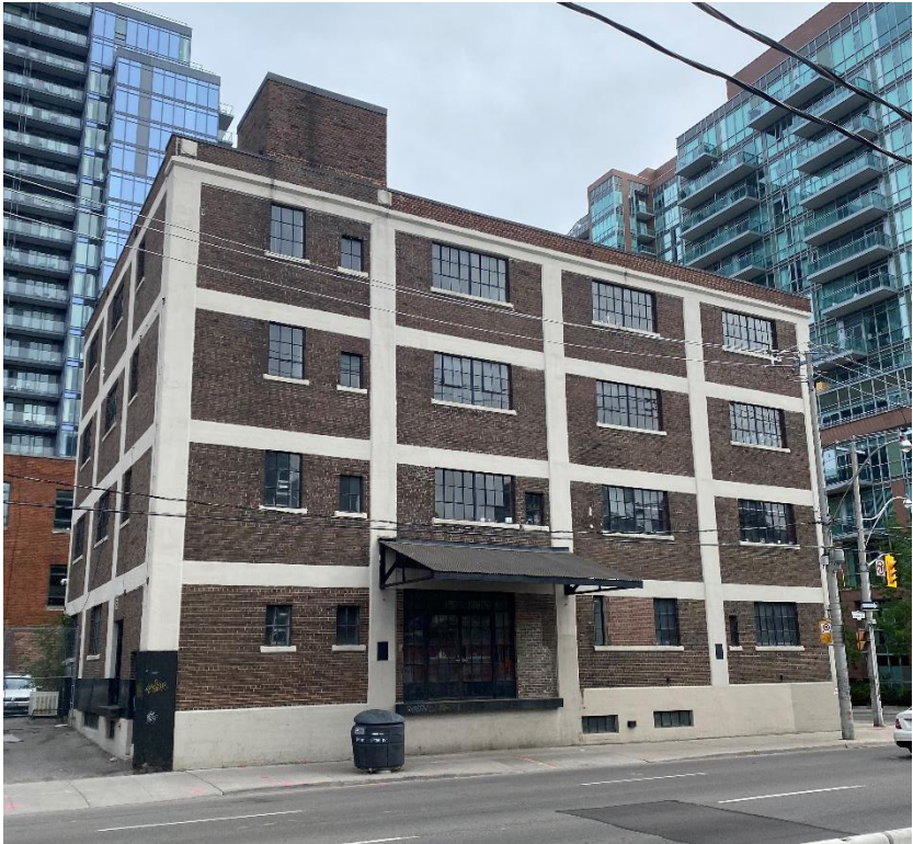
Figure 18: Current photo looking south and showing the north elevation of 125 George Street with its original loading bay and steel awning. (Heritage Planning, 2021)
