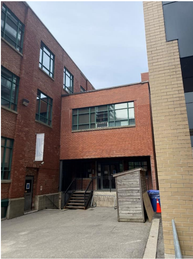
Figure 11: Current photo looking east and showing the 1950 one-storey addition to the Frankel Building complex. (Heritage Planning, 2021)
