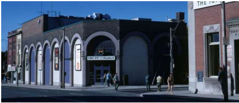
10. 1971 archival photograph showing the closed in arcade during the building's time as a film production studio for the CBC. The cast stone cornice and other decorative details are missing by this point. At left is the adjacent commercial row at 1130-1134 Yonge Street. (CoT Archives)
