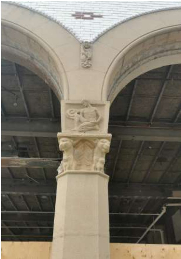
21. Detail of a cast stone arcade column with decorative sculptural detailing by artist, Merle Foster. (Heritage Planning, 2021)
