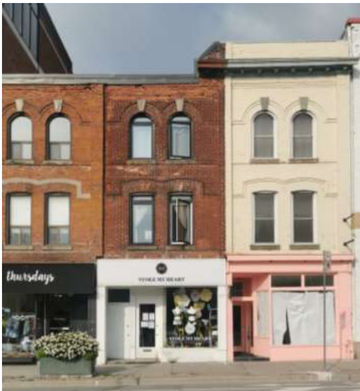
14. Current photograph of the principal (east) elevations of 1130-1134 Yonge showing the openings, the brick and stone detailing and the loss of the roof cornice and parapet at 1130 and 1132. (Heritage Planning, 2021)
