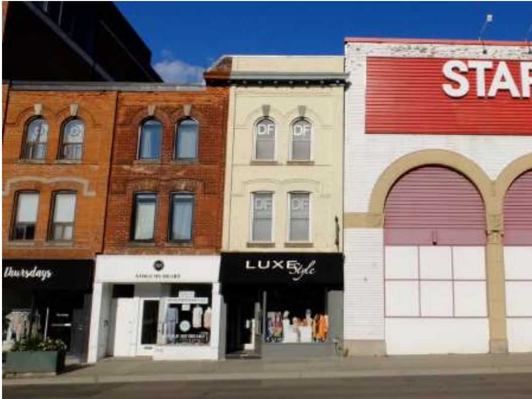
East elevation of the main street commercial row at 1130-1134 Yonge Street with part of the adjacent property at 1140 Yonge visible at right (ERA, 2020)
