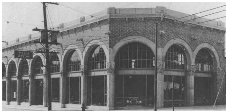
9. 1930 archival photograph of the recently completed Pierce-Arrow showroom. Note the projecting gargoyles in the arcade spandrels, now lost. (CoT Archives)
