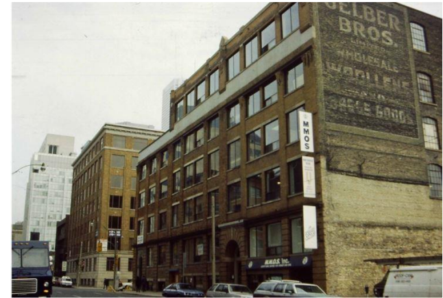
Gelber Building Addition, 1923, right New Textile Building, 1923 (photo, 1991)
