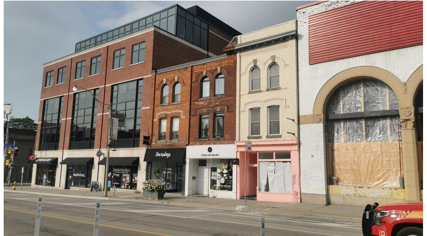
Current photographs of the principal (east) elevations of 1130-1134 Yonge Street showing the openings, the brick and stone detailing and the loss of the roof cornice and parapet at 1130 and 1132. [Heritage Planning, 2021]
