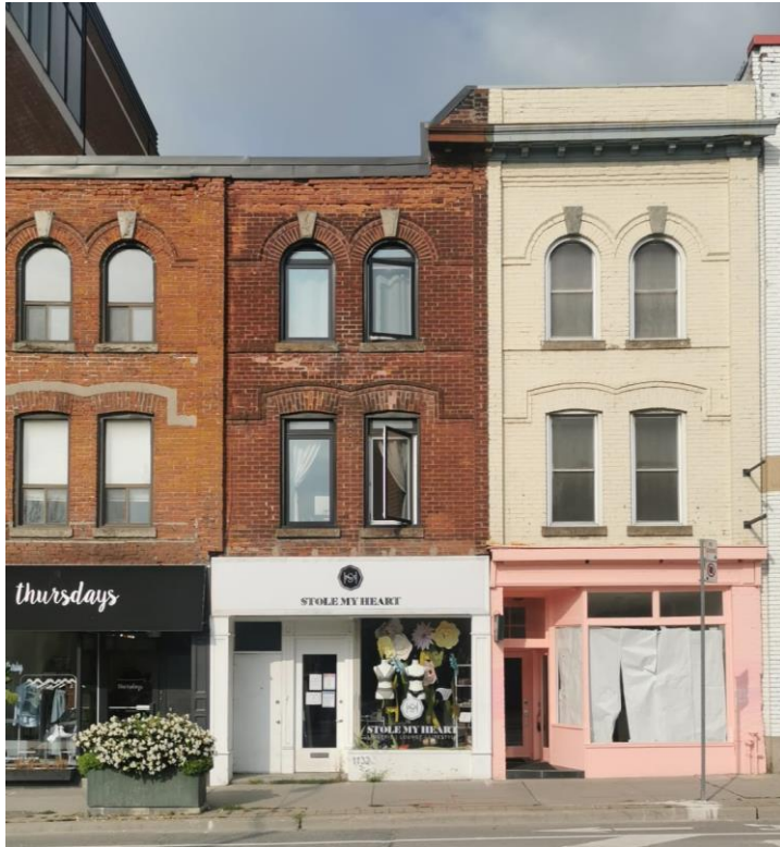
Current photographs of the principal (east) elevations of 1130-1134 Yonge Street showing the openings, the brick and stone detailing and the loss of the roof cornice and parapet at 1130 and 1132. [Heritage Planning, 2021]
