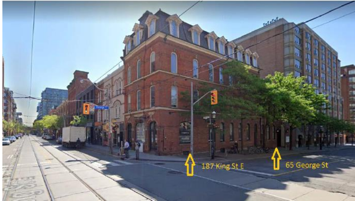
View looking south east
