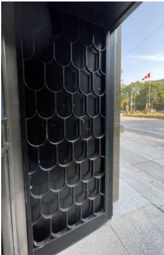
Figure 27: 250 University Avenue, east façade, security grill detail. Heritage Planning, 2021.
