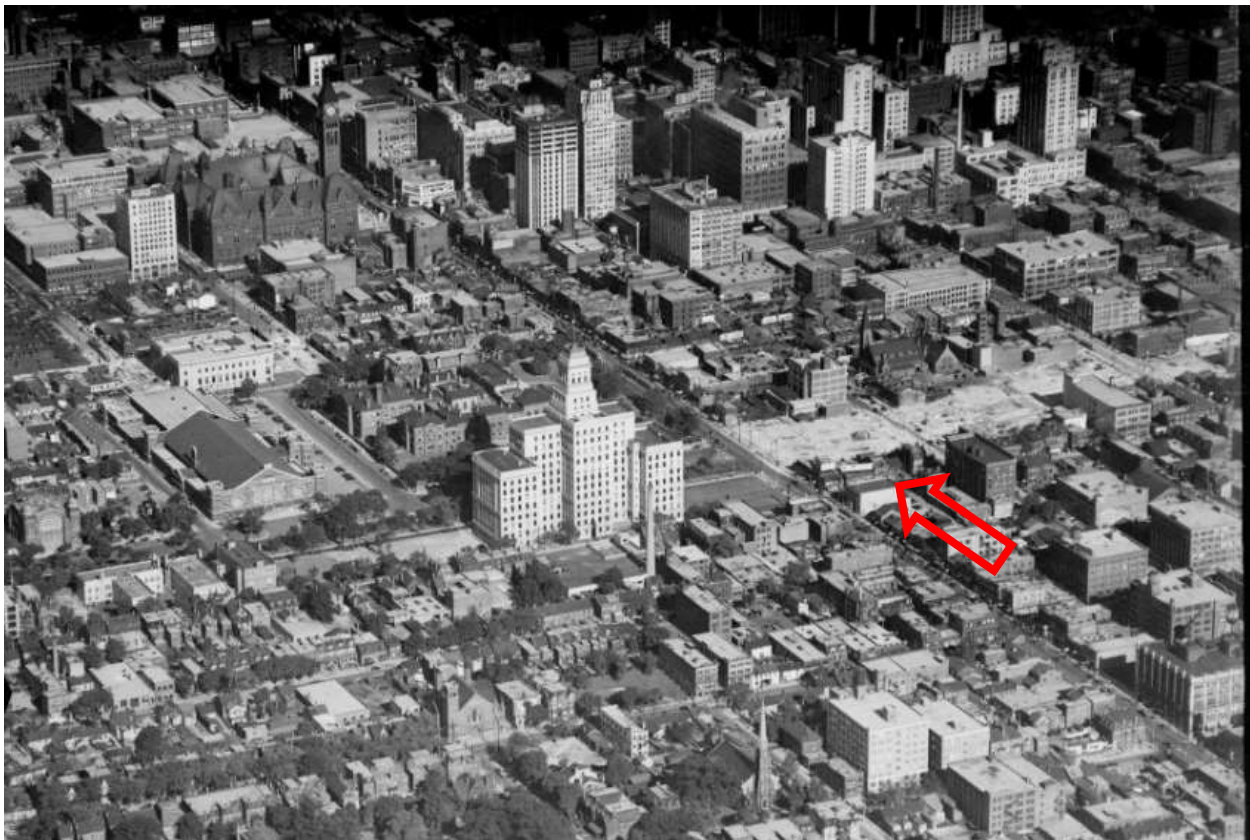
Figure 3: Aerial view of downtown from the northwest, showing the path of demolition prior to the extension of University Avenue south of Queen Street West, 1930 (City of Toronto Archives, fonds 1233, item 10092)
