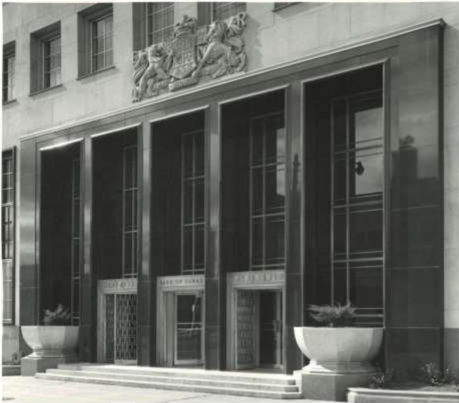
Figure 14: Toronto Agency main entrance – 250 University Avenue. ca. 1960. Photo: Panda Photography. Bank of Canada Archives (PC 315.2-92)
