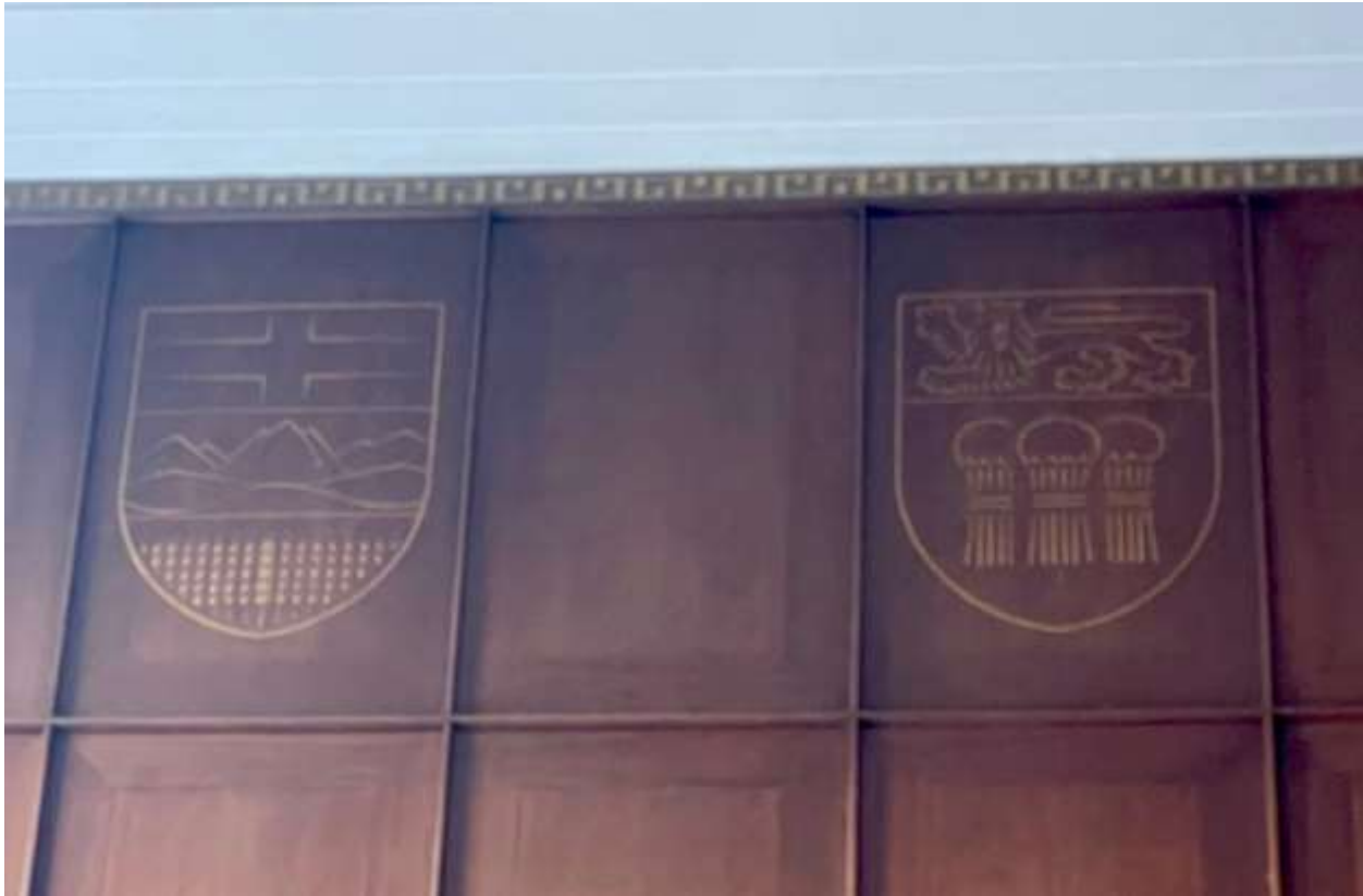
Figure 25: 250 University Avenue, entrance lobby, provincial crests with gold leaf gesso meander detail. Heritage Planning, 2021.
