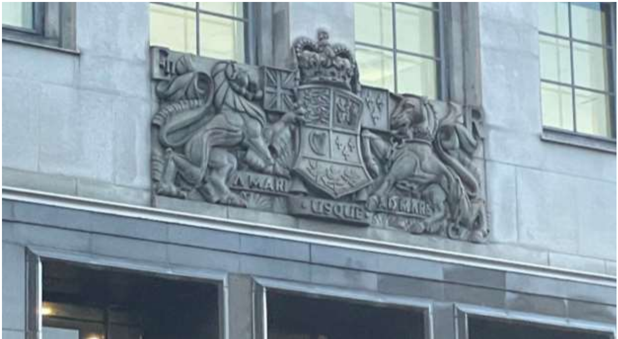
Figure 22: 250 University Avenue, east façade, coat of arms detail. Heritage Planning, 2021.
