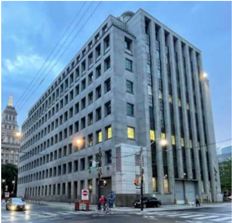
Figure 19: 250 University Avenue, south and west facades. Heritage Planning, 2021.
