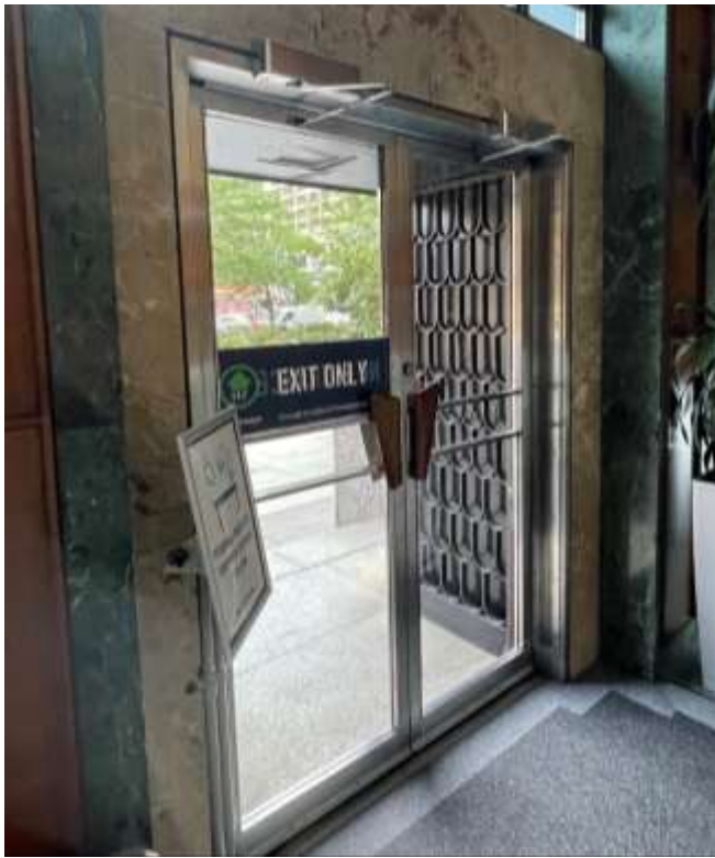
Figure 26: 250 University Avenue, entrance lobby, double doors. Heritage Planning, 2021.
