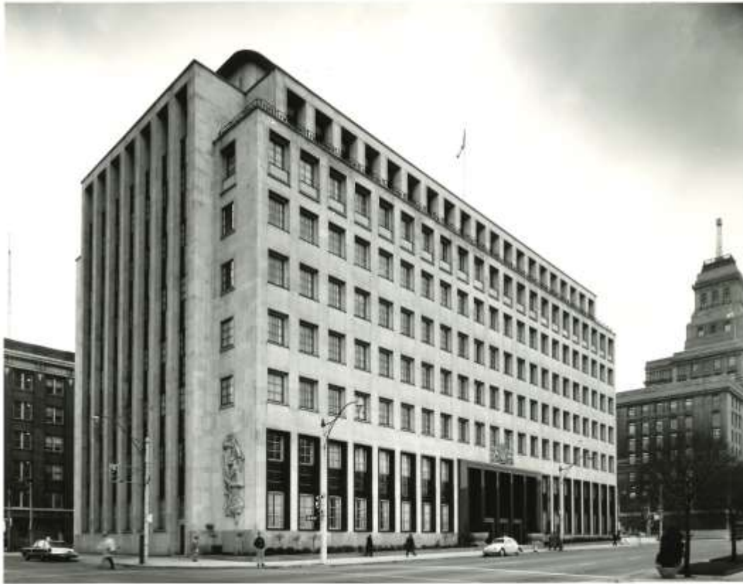
Figure 10: Toronto Agency south and eastern façades – 250 University Avenue. ca. 1960. Photo: Panda Photography. Bank of Canada Archives (PC 315.2-101)
