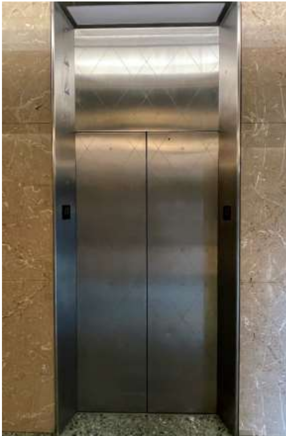
Figure 29: 250 University Avenue, elevator lobby, elevator door detail. Heritage Planning, 2021.
