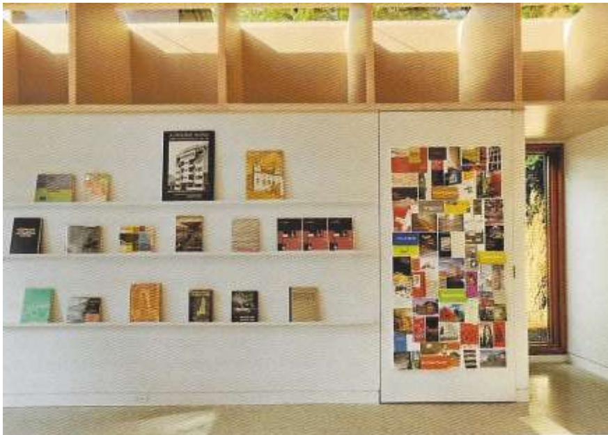
Figure 61. Studio Interior, north wall showing the deep coffers and their broad spacing with the display shelving below and the single window with a view of the rear garden and providing cross ventilation. (Photo credit: Bob Gundu, RAIC, Architecture Canada 2010: Governor General's Medals , p. 93.)
