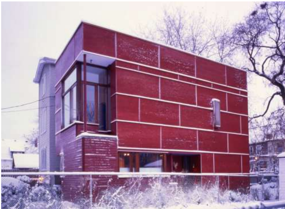
Figure 39. Craven Road House, west and south elevations with the effects of snow (Photo credit: Robert G. Hill)
