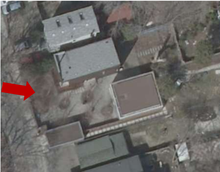
Figure 34. Aerial View of the property dated 2009 showing the house with the new studio, the courtyard with the planted circular planting beds for the river birches, the new garage for the neighbours and the new footpath. (City of Toronto Mapping, 2021)
