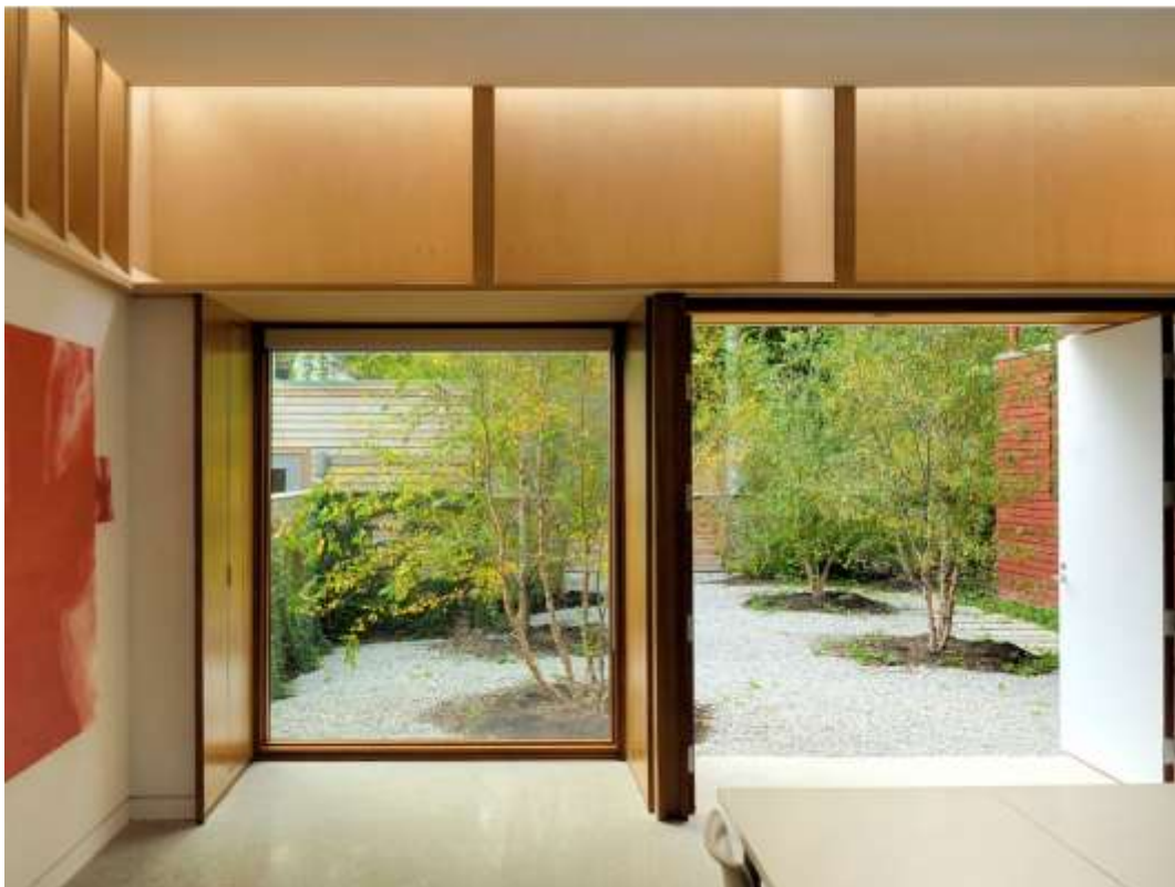
Figure 62. Studio interior looking west towards the landscaped courtyard with the bay window and panelled ventilation opening on the left, the double doors for a future garage function open. The coffers on this elevation are the furthest apart corresponding to the depth of the bays below. (Photo credit: Bob Gundu, RAIC, Architecture Canada 2010: Governor General's Medals , p. 90.)
