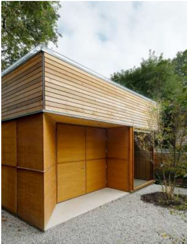
Craven Road Studio, 2004-6, Principal West elevation (Bob Gundu, RAIC, Architecture Canada 2010: Governor General's Medals , p.91)
