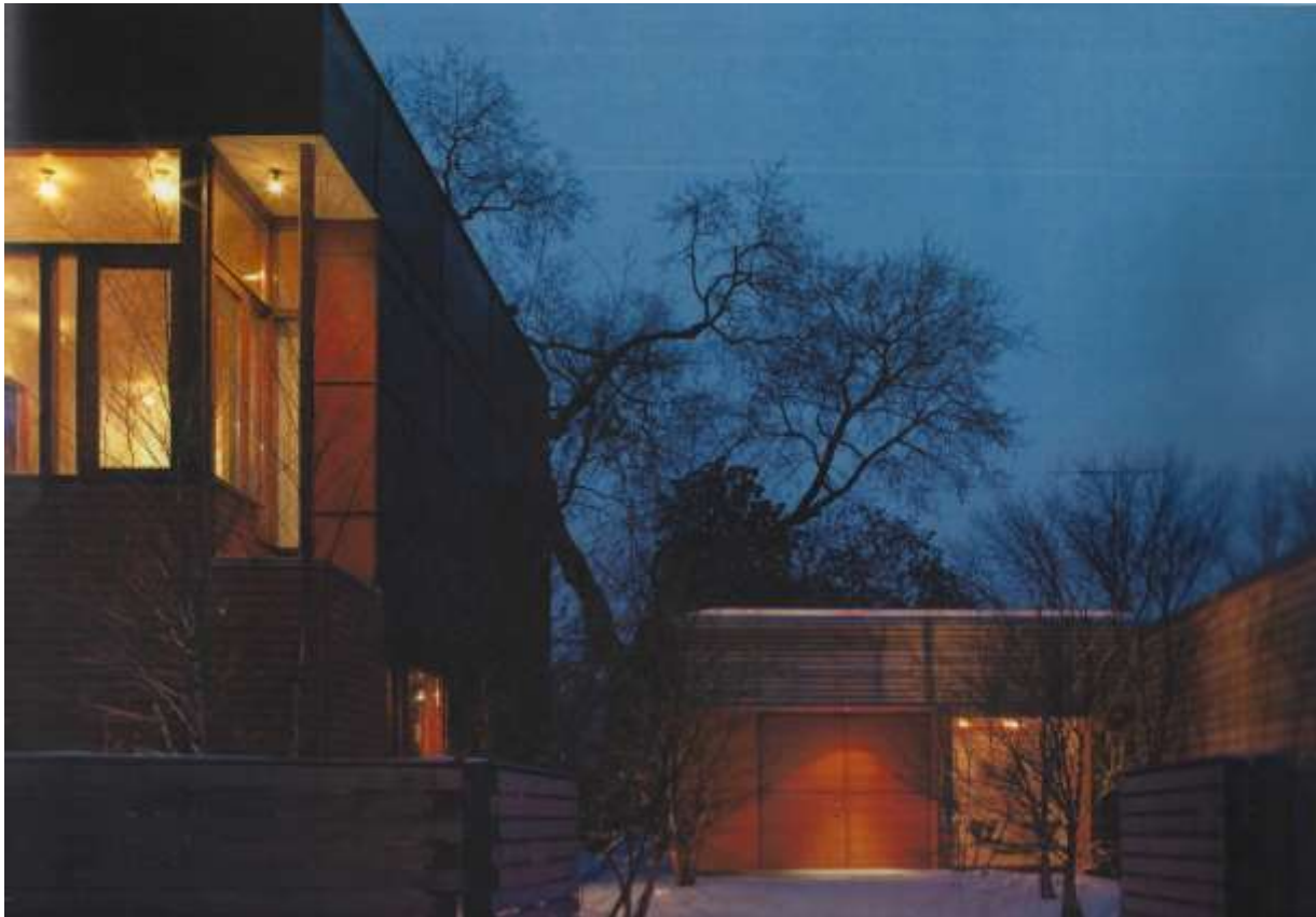
Figure 64. Winter View of the courtyard with the house and studio. (Photo credit: Steven Evans, provided by Shim-Sutcliffe Architects Inc.)
