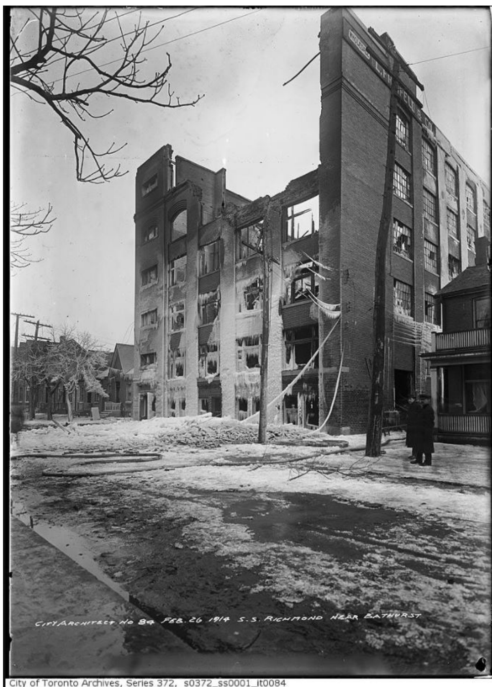
33. City Architect photograph "South side Richmond near Bathurst," No. 84, date February 26, 1914 of the Independent Cloak Co. building, on the south side of Richmond near Bathurst. The photograph shows that the original building was built as five-and-a-half storeys, departing from the drawings by adding an additional floor to the mid-section. Remnants of the original Chicago-style windows remain on the principal elevation facing Richmond Street with steel factory sash glazing on the west side elevation. The signage at the top says "Wholesale, L. Freifeld & Co." Louis Freifeld was recorded as a furrier and tenant with one of the two largest rental spaces as he occupied two of the upper floors of the building in the assessment rolls recorded on August 29, 1913. (City of Toronto Archives, Series 372, s0372, ss001,it0084)
