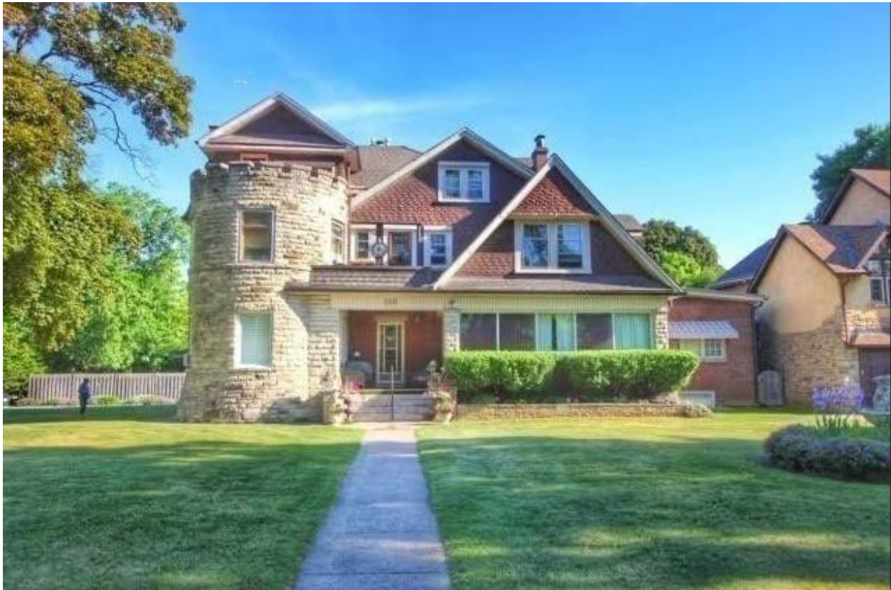
Principal (south) elevation of 180 Queens Drive (House Sigma)
