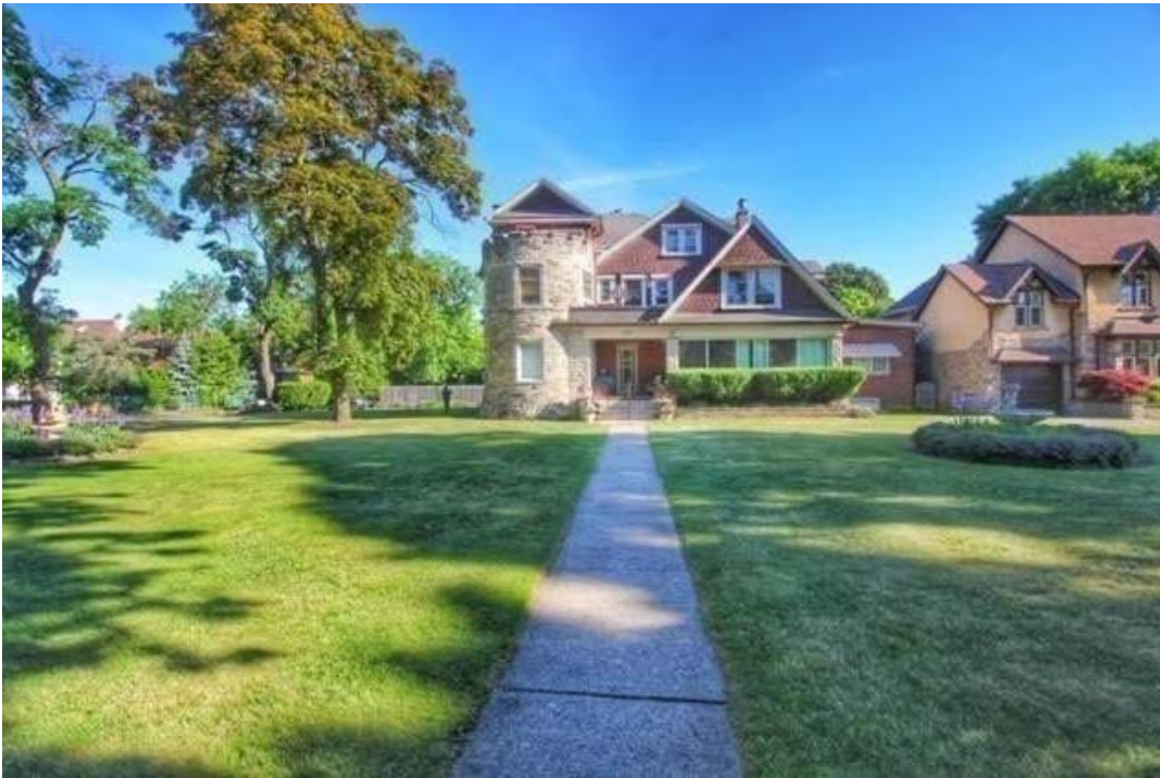
Figure 8. Principal (south) elevation of 180 Queens Drive (House Sigma)
