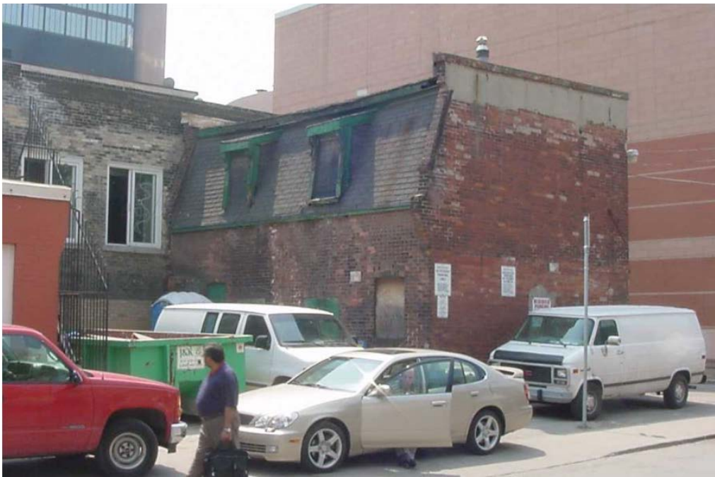
12. 2001 archival photograph, showing the rear coach house at 526 Yonge Street. Note this structure originally echoed the Second Empire design of the main building, featuring brick construction, and a mansard roof with shed-roofed dormers on brackets and parapet firewalls. (Heritage Planning, 2001)
