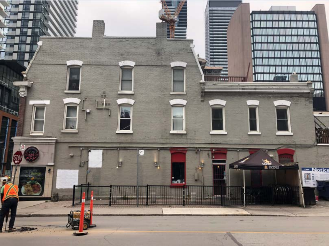
19. Current photo looking south from Breadalbane Street, showing the secondary (north) elevation of the building at 526 Yonge Street, located at the southwest corner of Yonge and Breadalbane Streets. (Heritage Planning, 2021)
