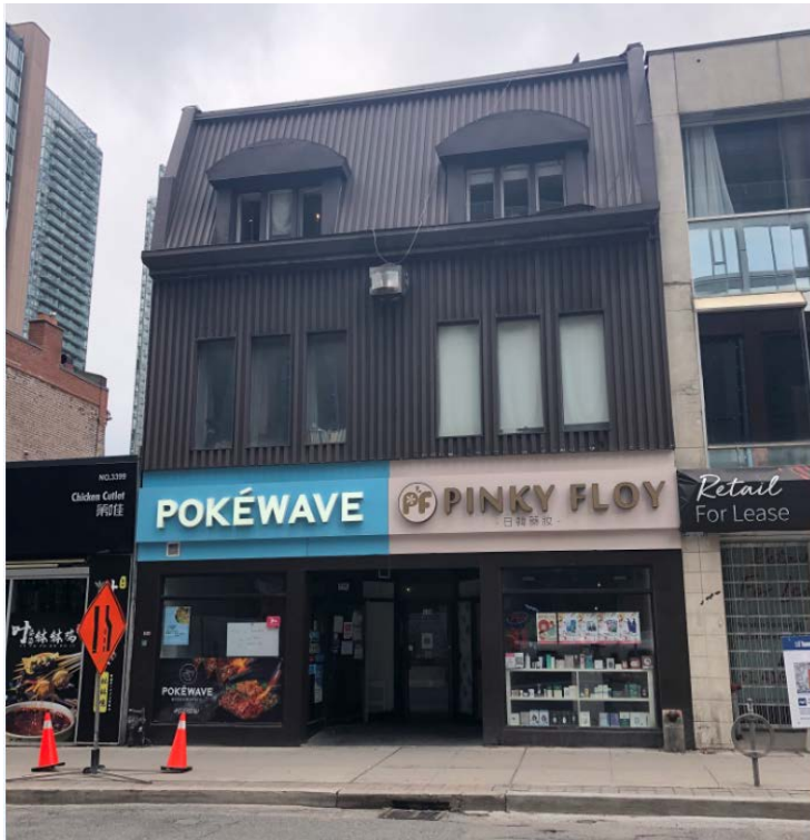
East (principal) elevation of 516 Yonge Street (Heritage Planning, 2021)
