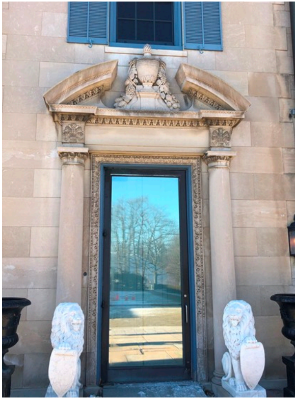
34. East elevation entrance from terrace (left)
