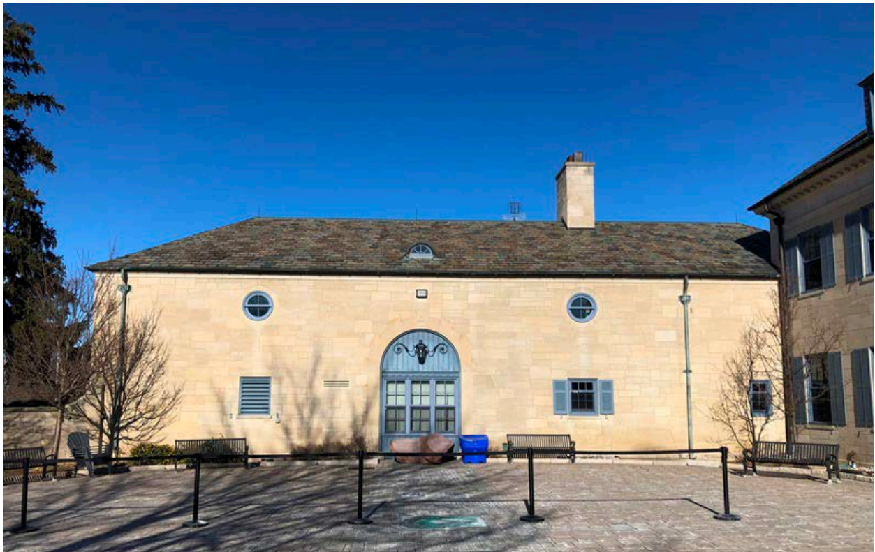
30. View of the service-garage building, south elevation
