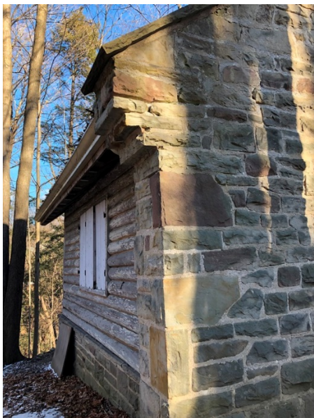
51. Corbel detail at the north-west corner of the cabin
