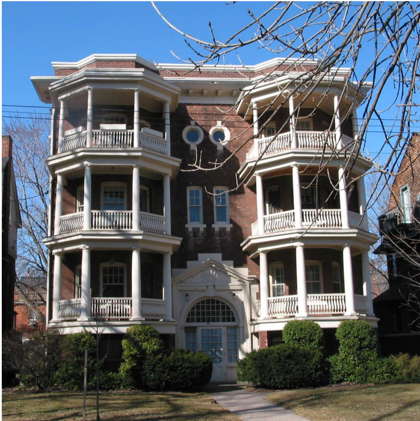
Figure 2: Principal (East) elevation of 68 Kendal Ave
