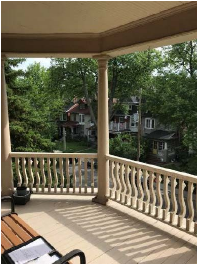
Figure 3: Typical view of balcony condition
