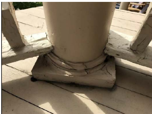
Figure 4-5: Deterioration at column bases
