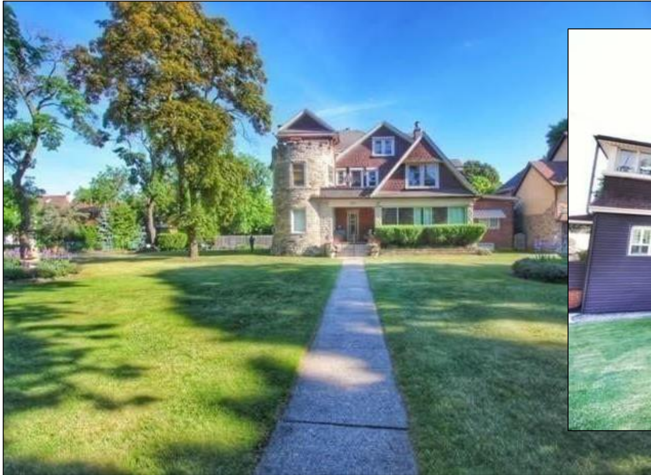
View of 180 Queens Drive looking northwest (House Sigma)
