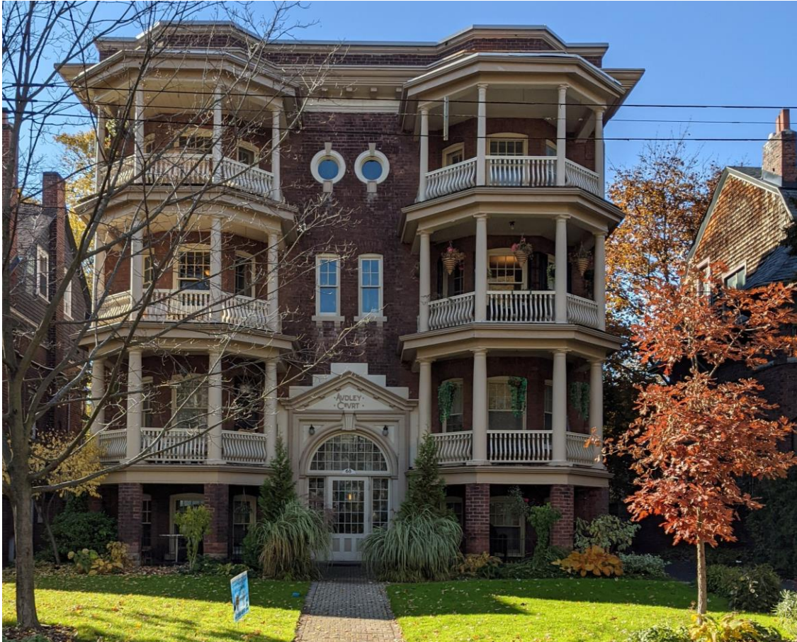
68 Kendal Avenue; Principal (East) elevation (Heritage Planning, 2021)
