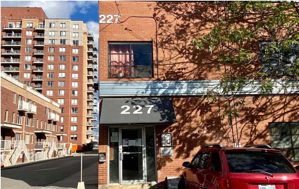
Figure 41: West elevation of the subject property's northern portion (dating to c.1954-1965), including the main entry to this part of the building. (Heritage Planning, 2021.)
