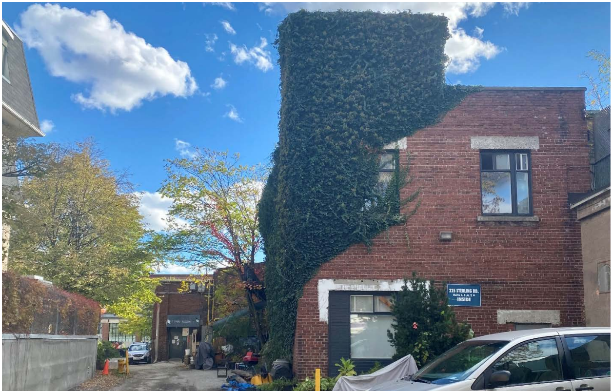
Figure 36: Southward view of a portion of the subject property's east elevation, dating to c.1924-1939. (Heritage Planning, 2021.)
