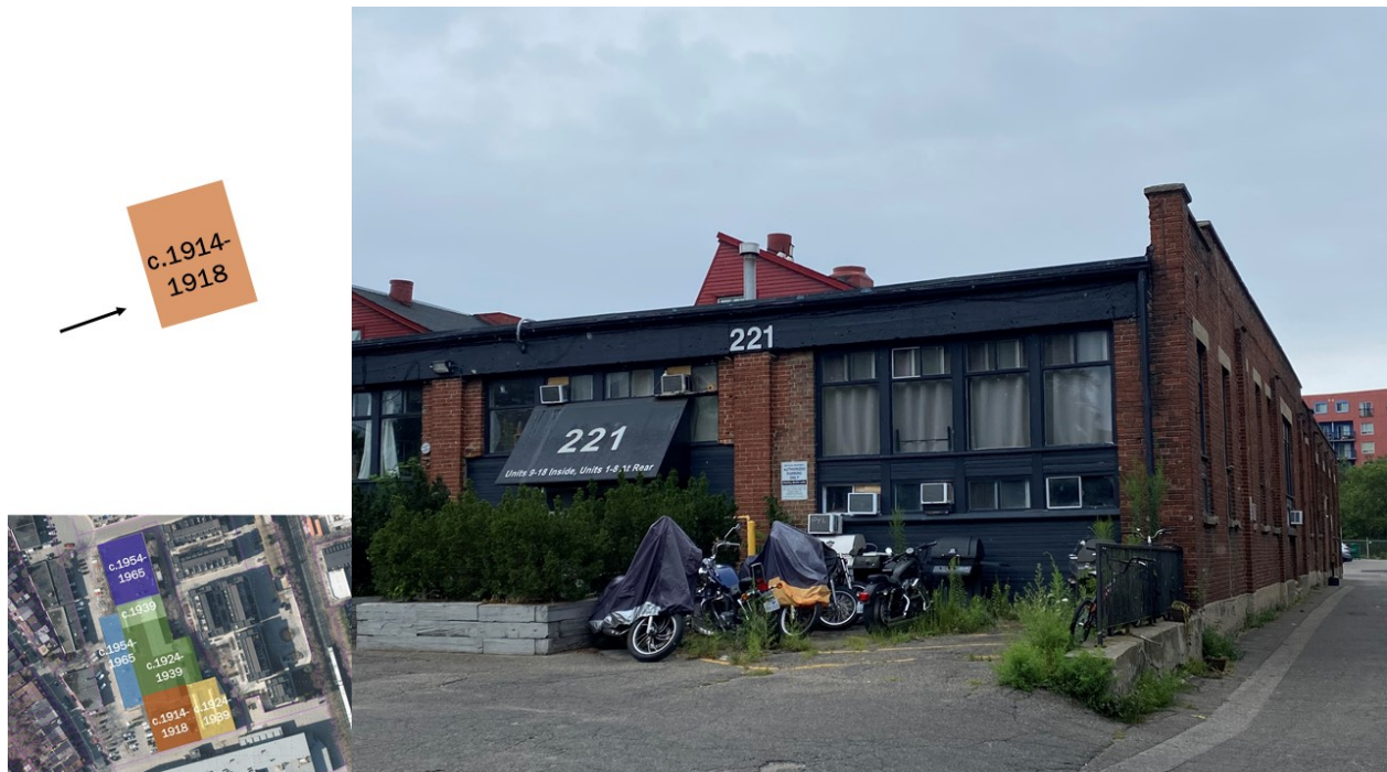
Figure 21: View of the c.1914-1918 portion of the building (with arrow indicating direction of view). (Heritage Planning, 2021.)
