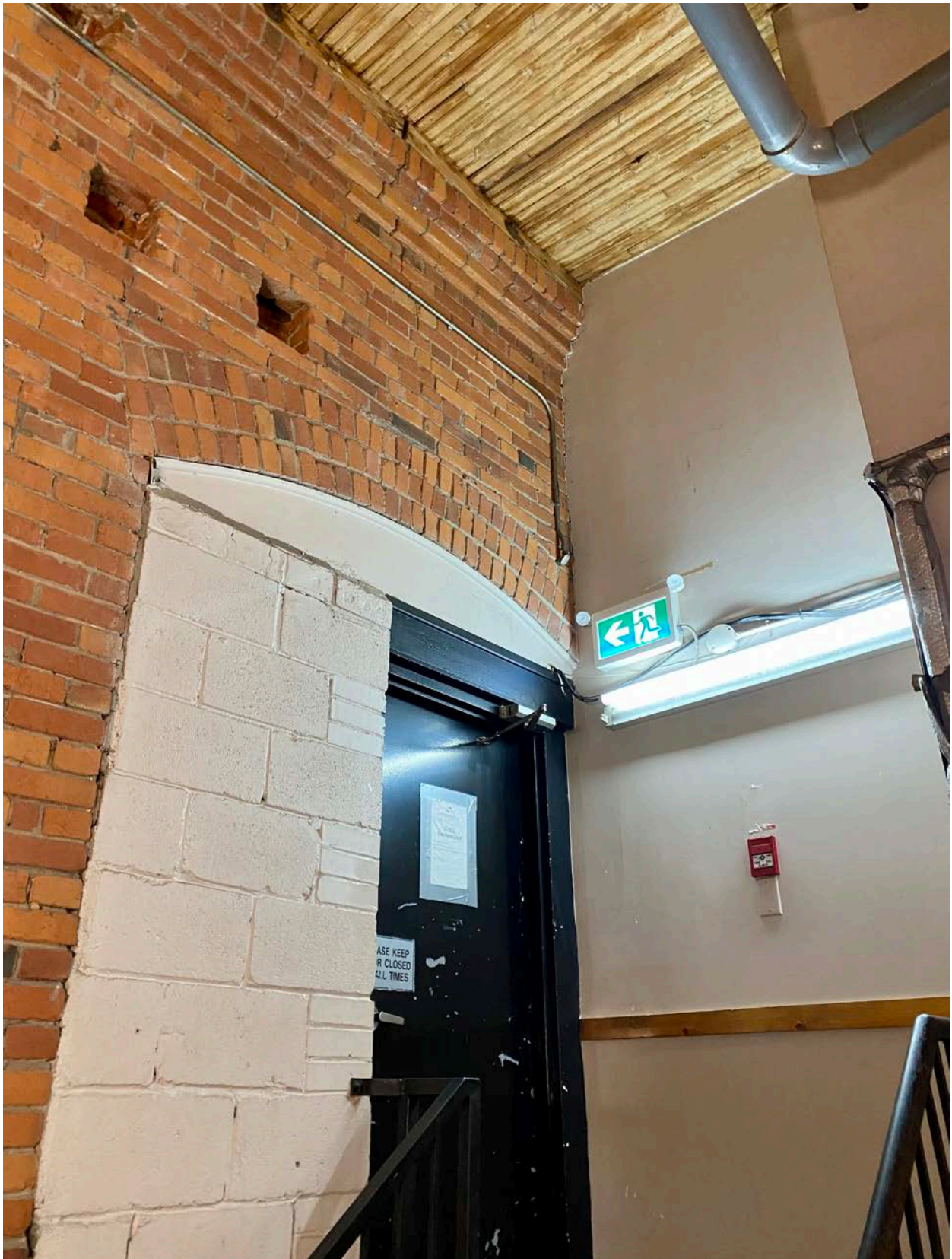
Figure 49: Interior of a fire escape door on the subject property's east elevation, within a portion dating to c.1939. (Heritage Planning, 2021.)
