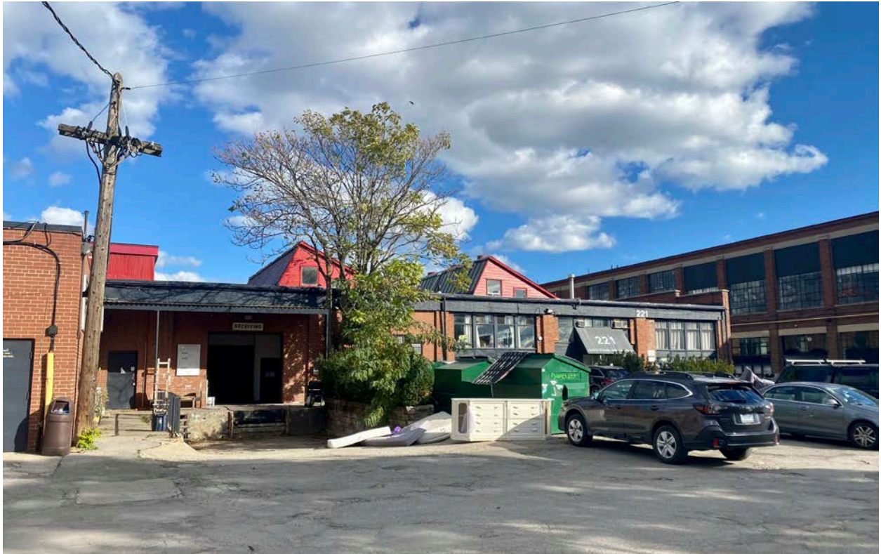
Figure 28: West elevation of the subject property's southwestern portion (dating to c.1914-1918). (Heritage Planning, 2021.)
