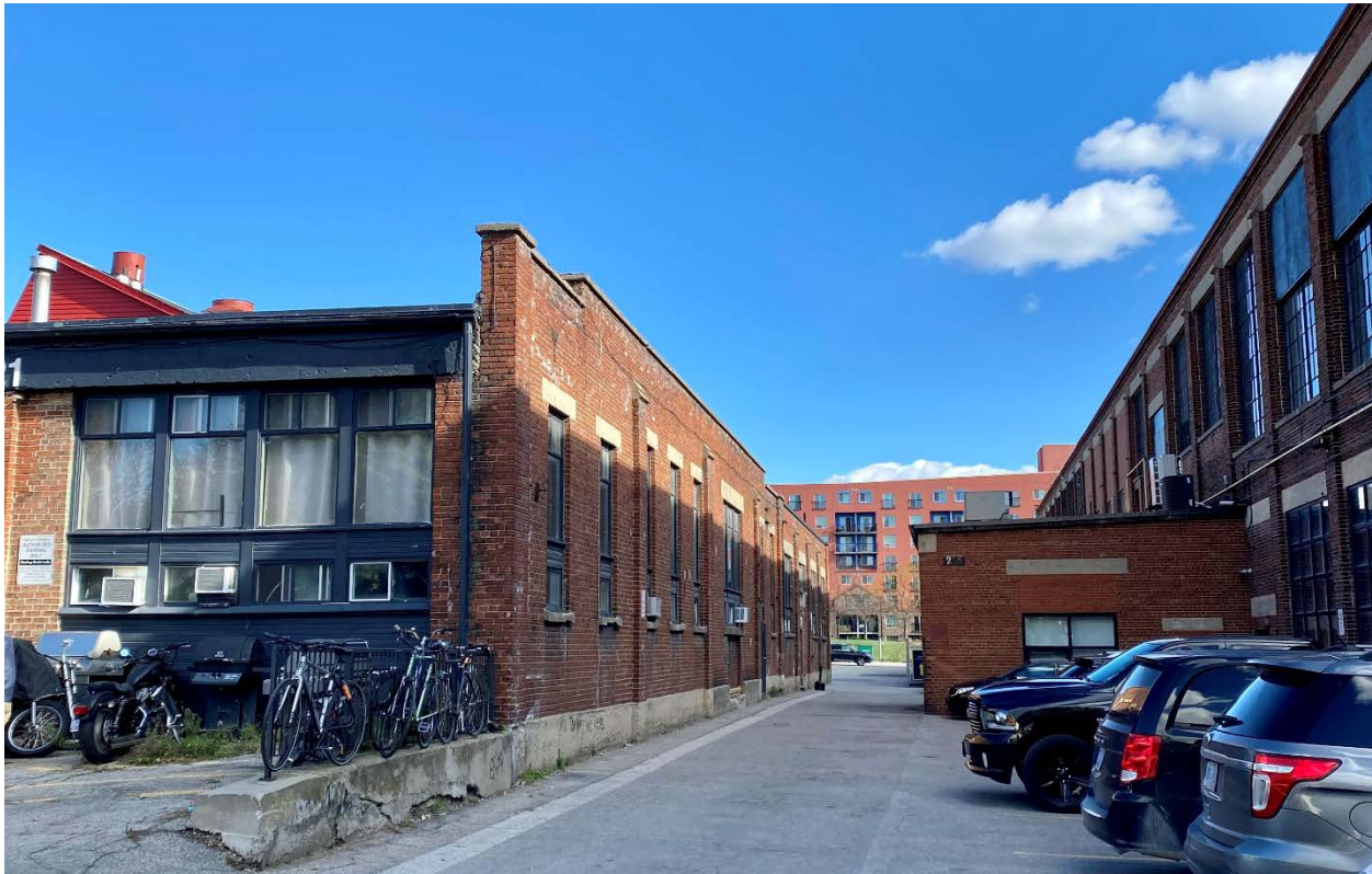
Figure 29: Eastward view of the alley formed by the subject property's south elevation and the north elevation of 213 Sterling Road. (Heritage Planning, 2021.)
