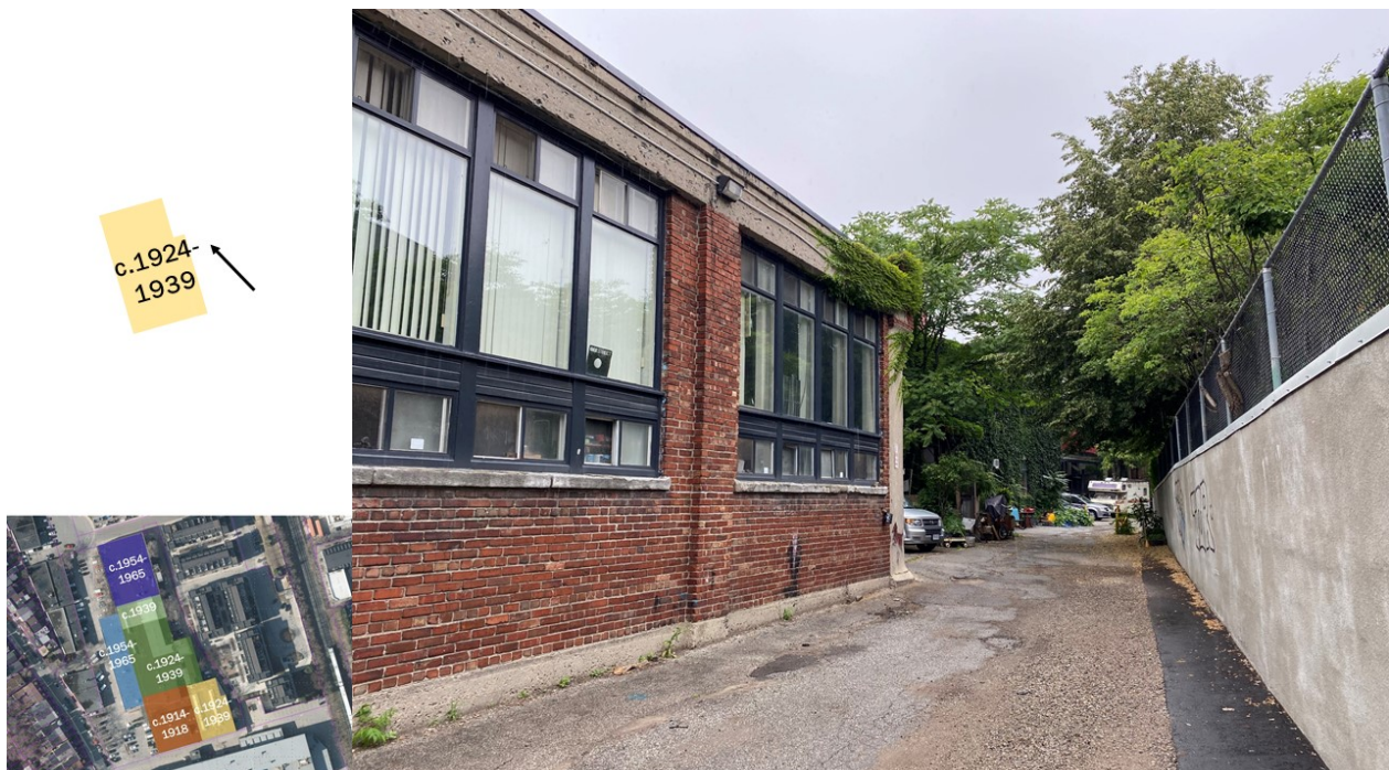
Figure 22: View of the southeastern c.1924-1939 portion of the building (with arrow indicating direction of view). (Heritage Planning, 2021.)
