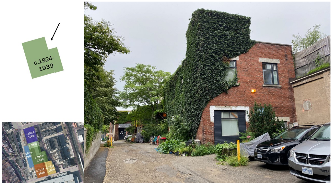
Figure 23: View of the central c.1924-1939 portion of the building (with arrow indicating direction of view). (Heritage Planning, 2021.)
