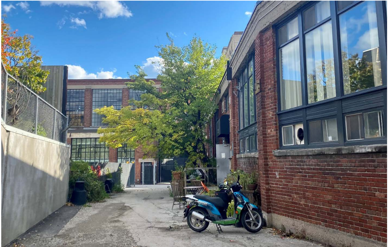
Figure 32: Southward view of a portion of the subject property's east elevation, dating to c.1924-1939, with 213 Sterling Road visible in the background. (Heritage Planning, 2021.)
