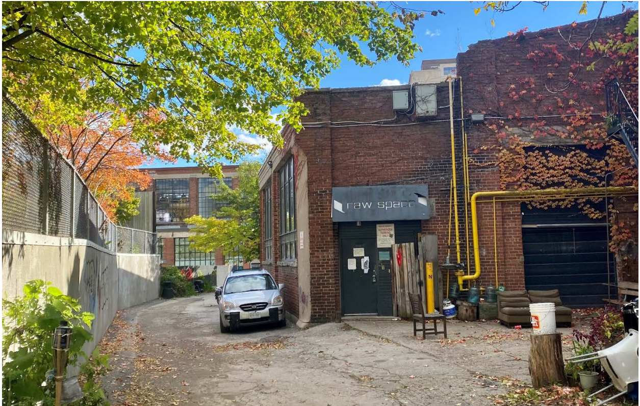
Figure 34: Southward view of a portion of the subject property's east elevation, dating to c.1924-1939. (Heritage Planning, 2021.)
