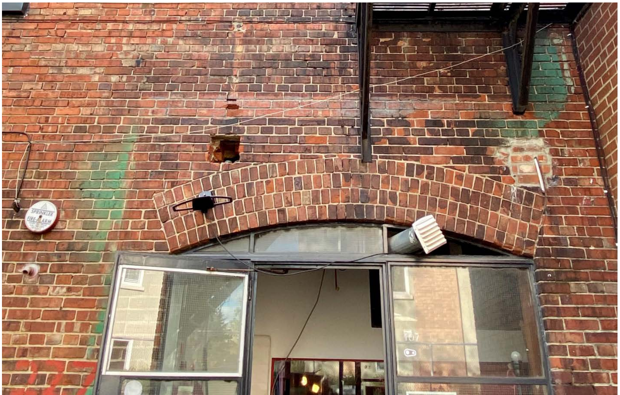
Figure 38: Upper level of the east elevation of an addition to the subject property, dating to c.1939, showing a brick row-lock arch. (Heritage Planning, 2021.)
