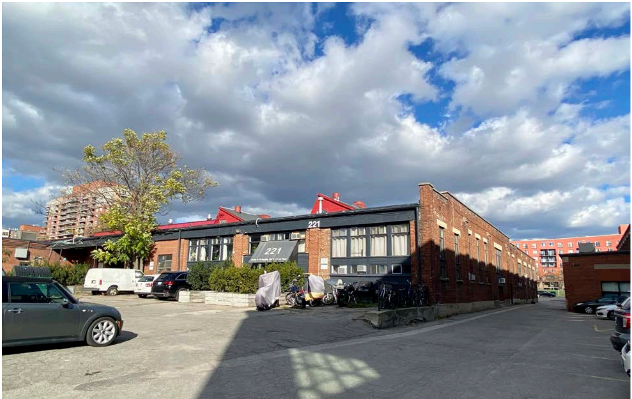
Figure 27: Northeastward view of the subject property's southwestern portion (dating to c.1914-1918). (Heritage Planning, 2021.)
