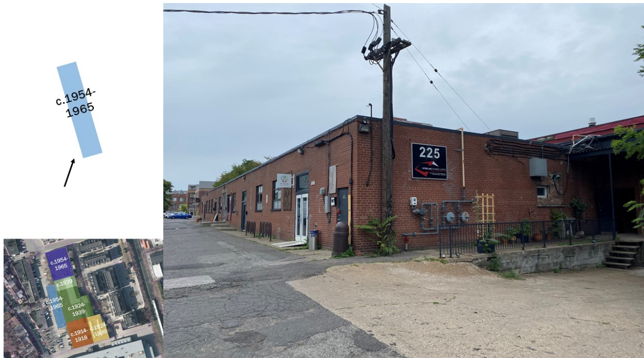
Figure 25: View of the western c.1954-1965 portion of the building (with arrow indicating direction of view). (Heritage Planning, 2021.)
