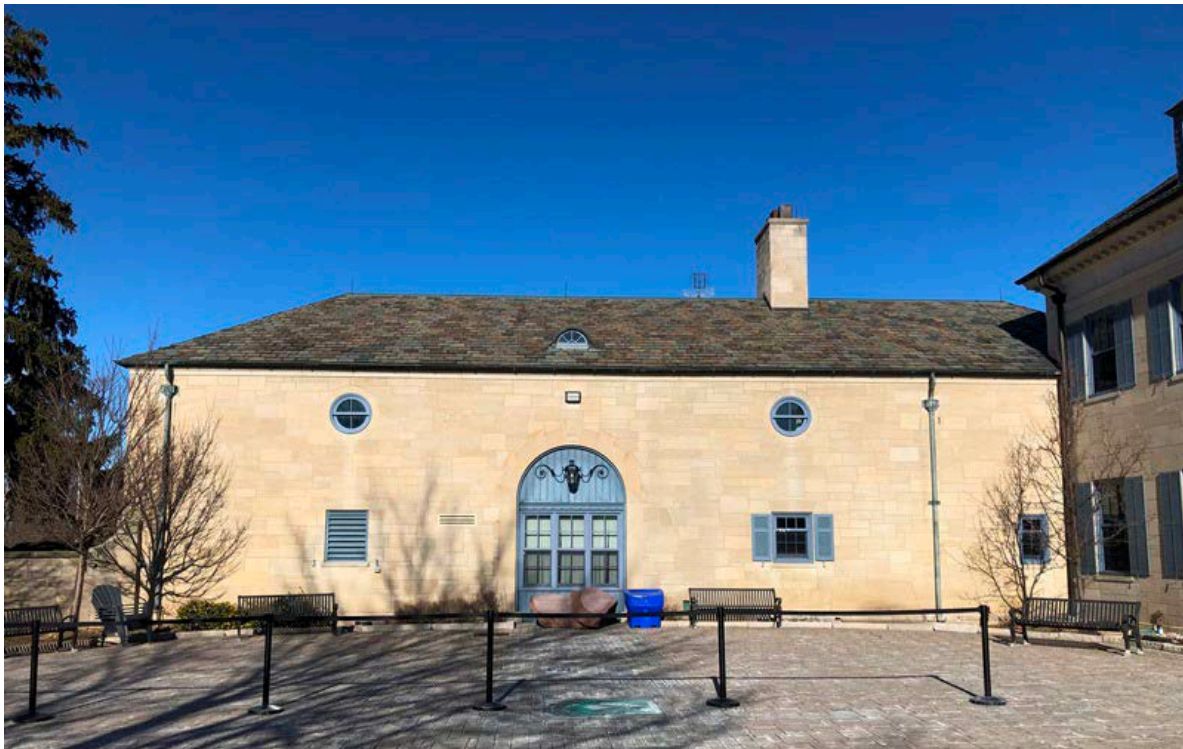
4. View of the service-garage building, south elevation
