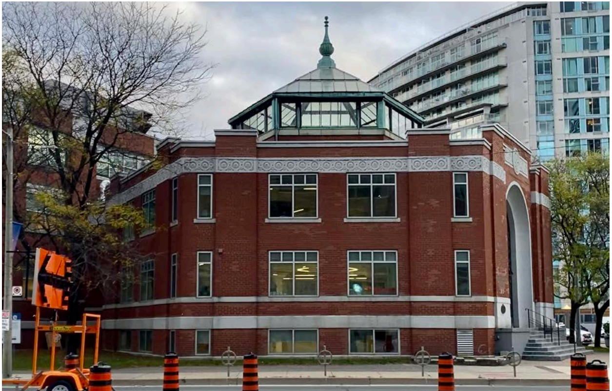
Figure 36: 545 Lake Shore Boulevard West; view of the hexagonal pavilion's north elevation. (Heritage Planning, 2021.)
