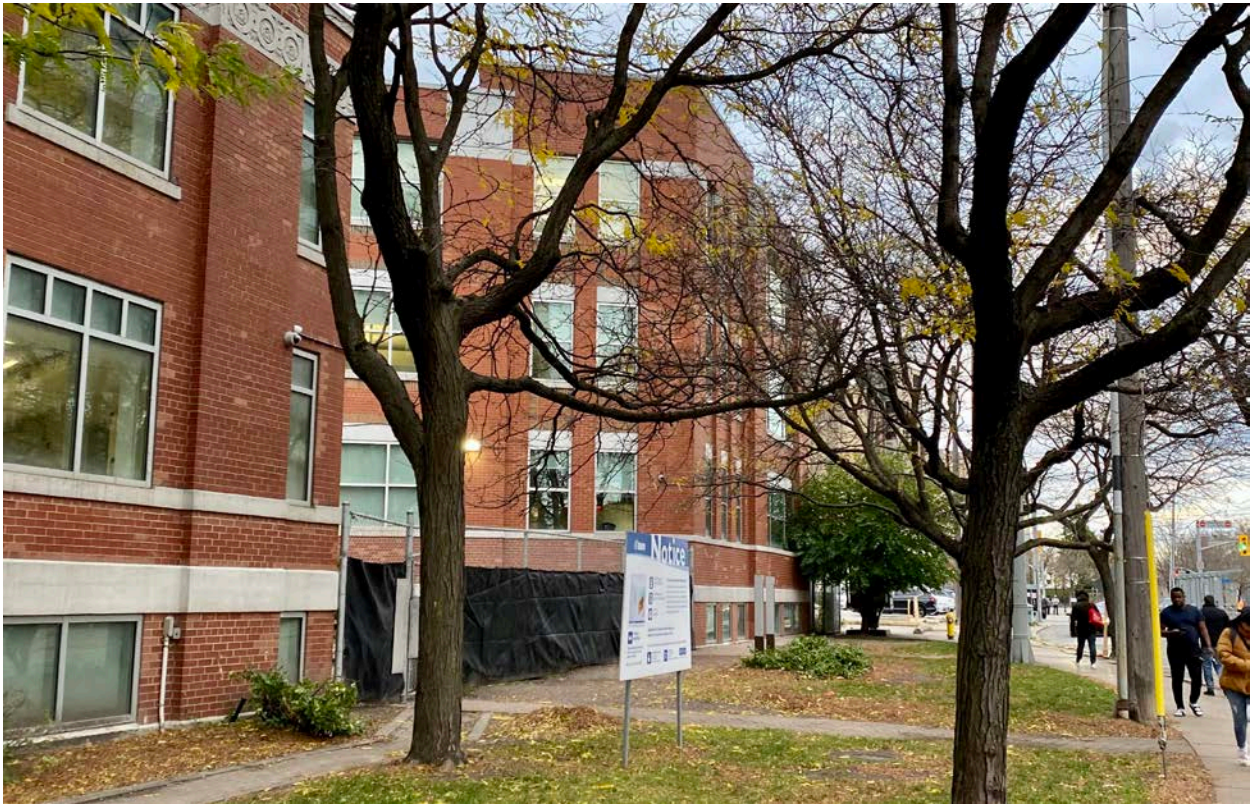
Figure 40: 545 Lake Shore Boulevard West; southward view along Bathurst Street. (Heritage Planning, 2021.)
