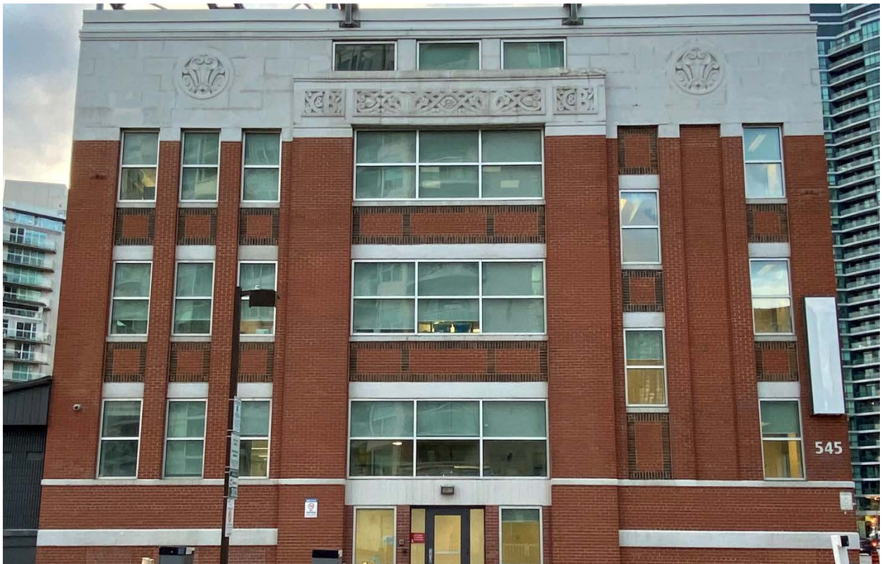
Figure 44: 545 Lake Shore Boulevard West; east elevation of the building's northeast wing. (Heritage Planning, 2021.)
