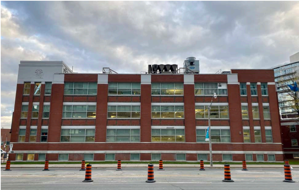
Figure 37: 545 Lake Shore Boulevard West; view of the northeast wing's north elevation along Lake Shore Boulevard West. (Heritage Planning, 2021.)
