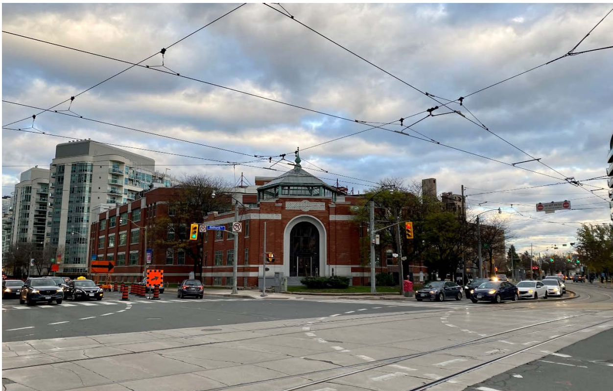
Figure 1: 545 Lake Shore Boulevard West; view of the property's northwest corner from the intersection of Lake Shore Boulevard West and Bathurst Street. (Heritage Planning, 2021.)
