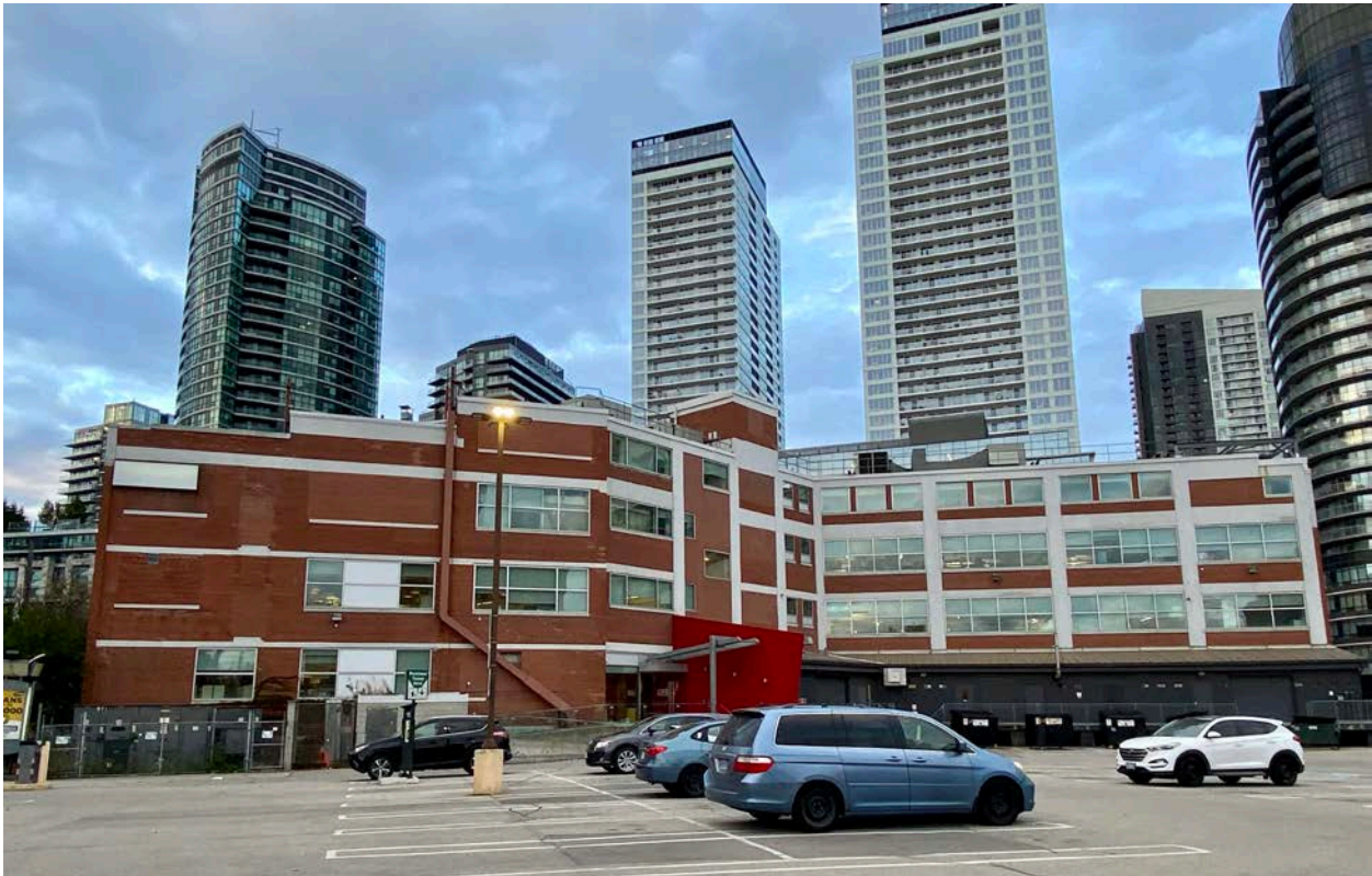
Figure 43: 545 Lake Shore Boulevard West; rear (south) elevation. (Heritage Planning, 2021.)
