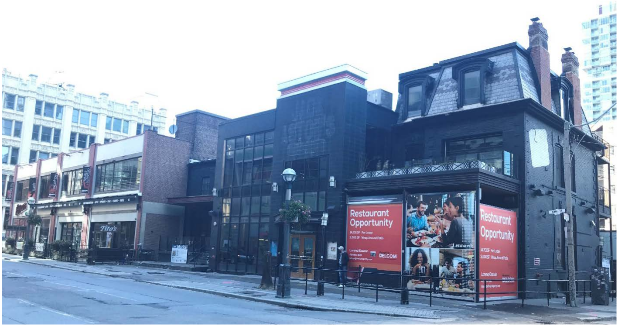
11. Contextual photograph looking northeast and showing the properties at (from left to right) 241 Richmond Street West and consolidated properties comprising 133 John Street. (Heritage Planning, 2021)
