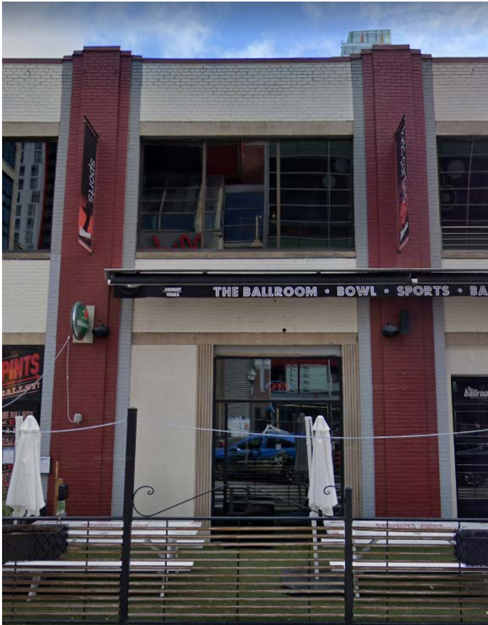
10. Current image showing a detail of the principal (west) elevation at 241 Richmond Street West with the original cast-stone, fluted door jamb and the stepped parapets that terminate the piers at the roofline. (Google, 2021)
