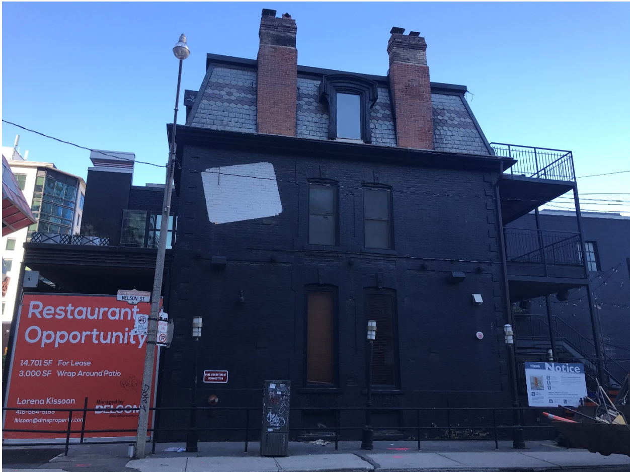
13. Current photograph showing the south elevation of 133 John Street fronting Nelson Street. The original openings, dichromatic brick chimneys, Mansard roof with slate tiles and decorative wooden roof dormers are all intact. (Heritage Planning, 2021)
