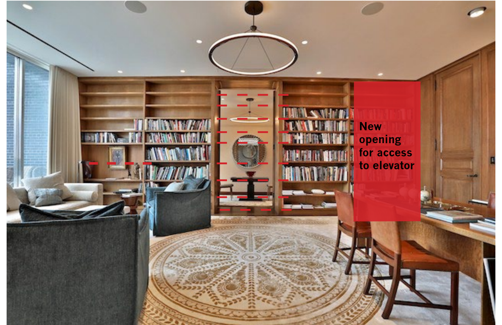
Permitted Alteration Schedule of the HEA for 130 Bloor St. W. (2) Interior (a). In the 13th Floor Library (Southwest corner), a new opening may be permitted to access a new room to the west. Restore the continuity of bookshelves as shown in Panda Associate's photo on the left.
