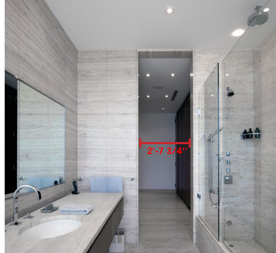
Photo of Current Southeast Bathroom, showing modifications to shower/tub on right side. New drywall ceiling, new shower fixtures and new glass enclosure were added. The recess for soap was removed. (ERA Architects / Steven Evans Photographer, 2020)
