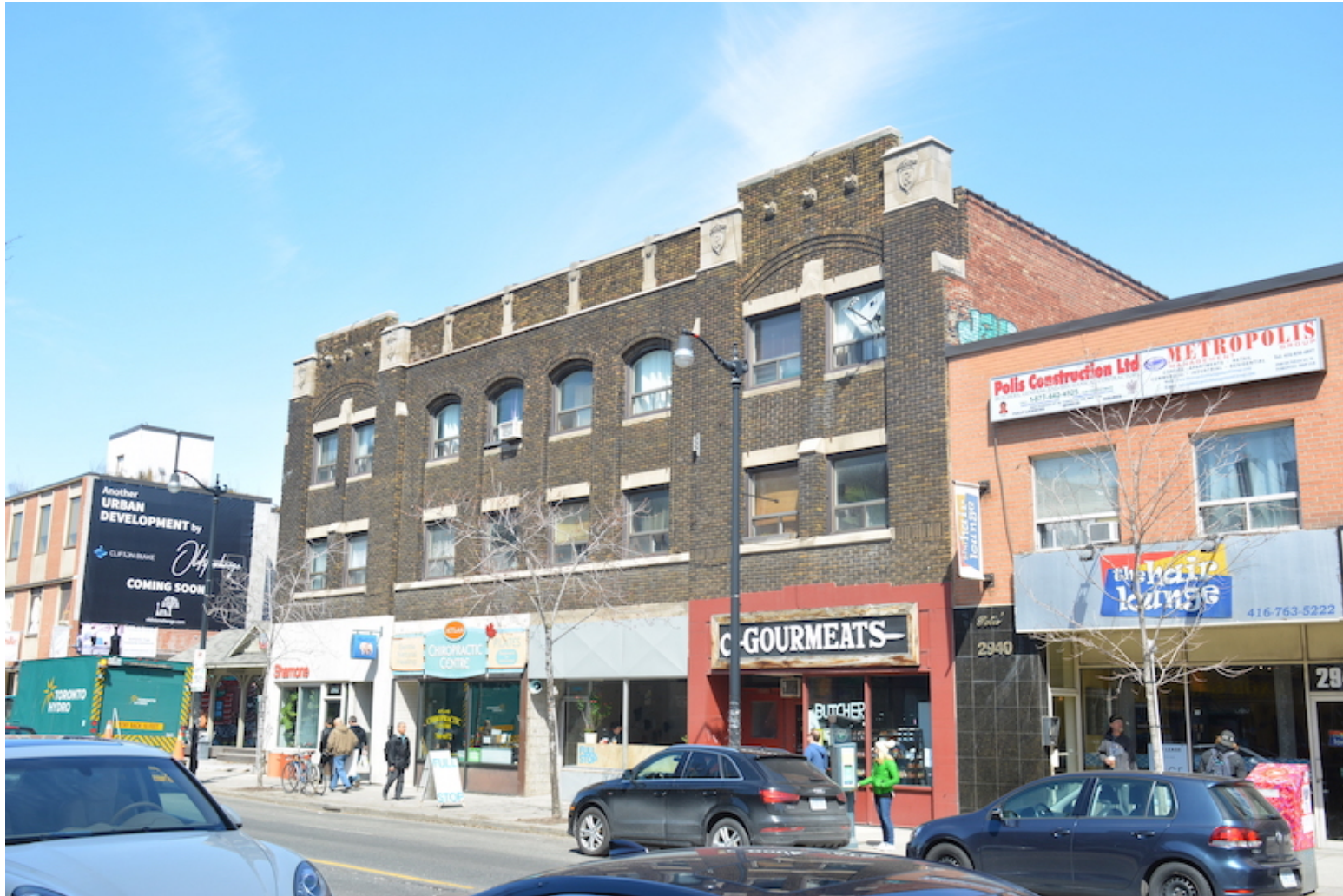
Dundas Street, looking northwest
