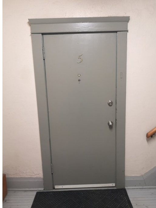
typical entrance door
