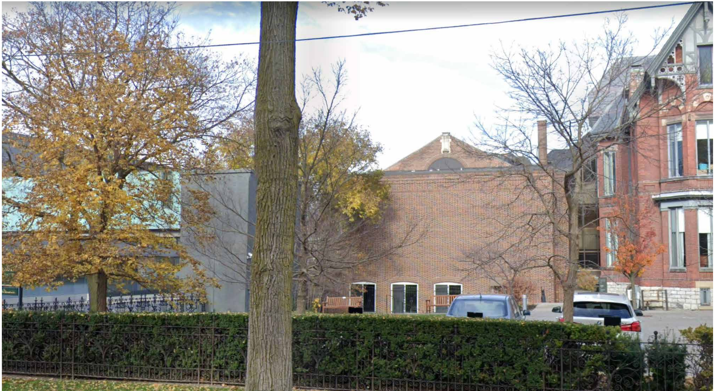
Context South Elevation of the 1978 addition
