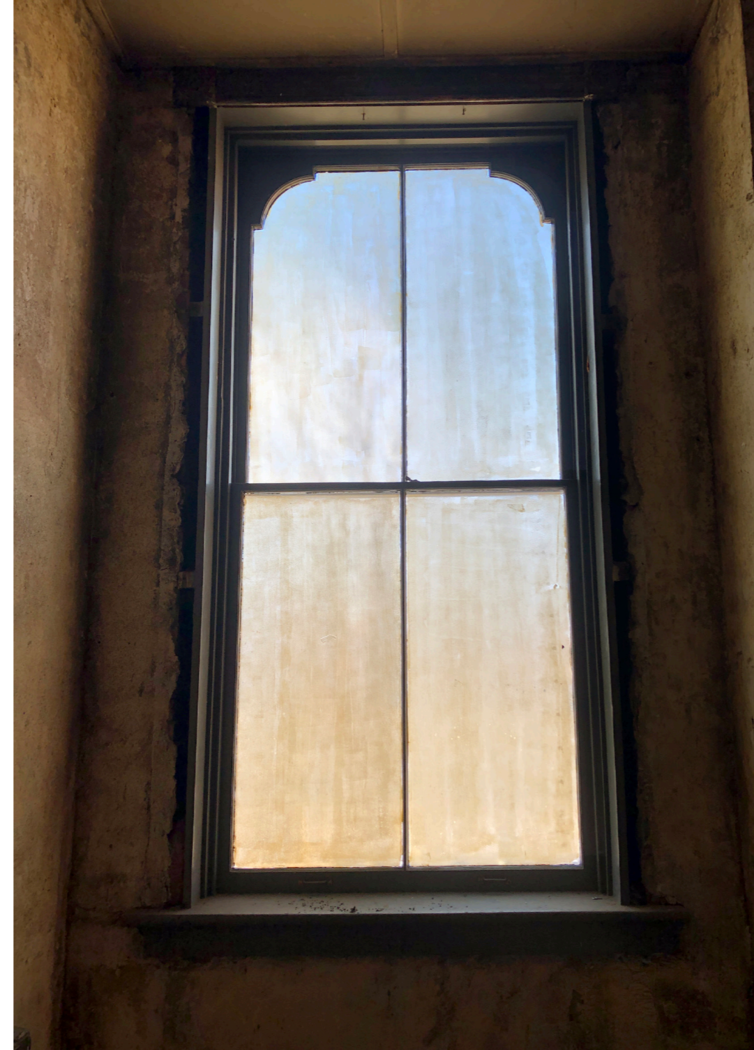
Window at school house to be rehabilitated. Photo from ERA
