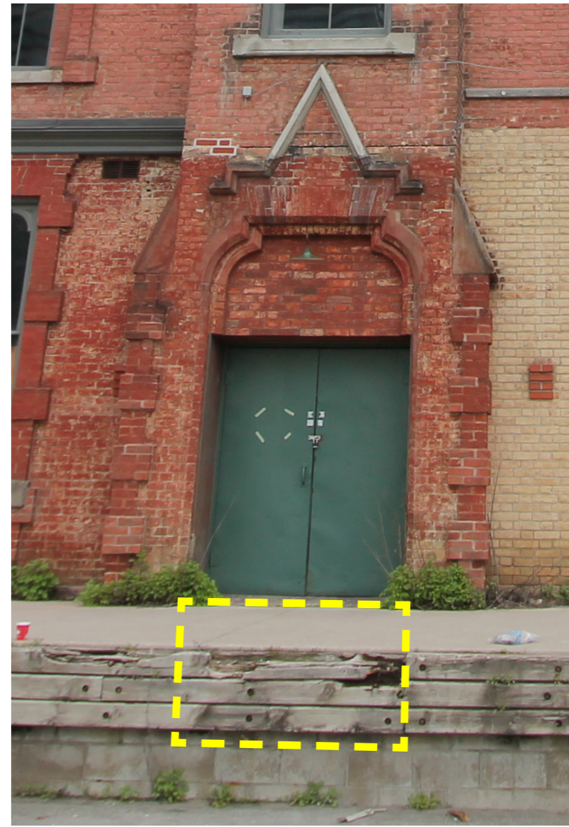
Lower existing sill to grade. Photo from ERA
