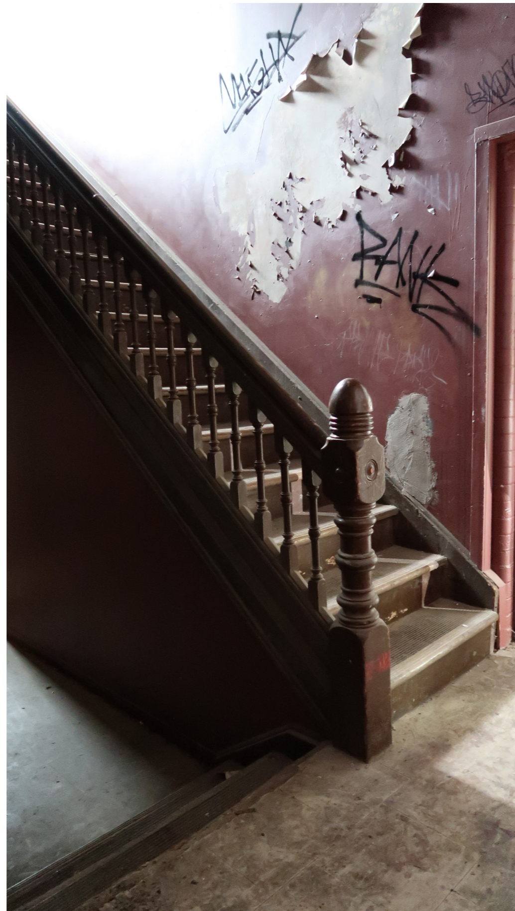
North heritage stair to be retained and rehabilitated. Photo by ERA
