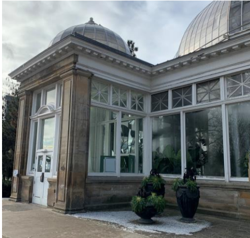
Exterior Elevation of an as-existing window bay.
