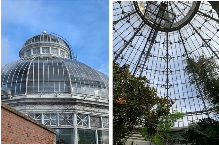
Exterior and interior view of the existing overhead plate glass.
