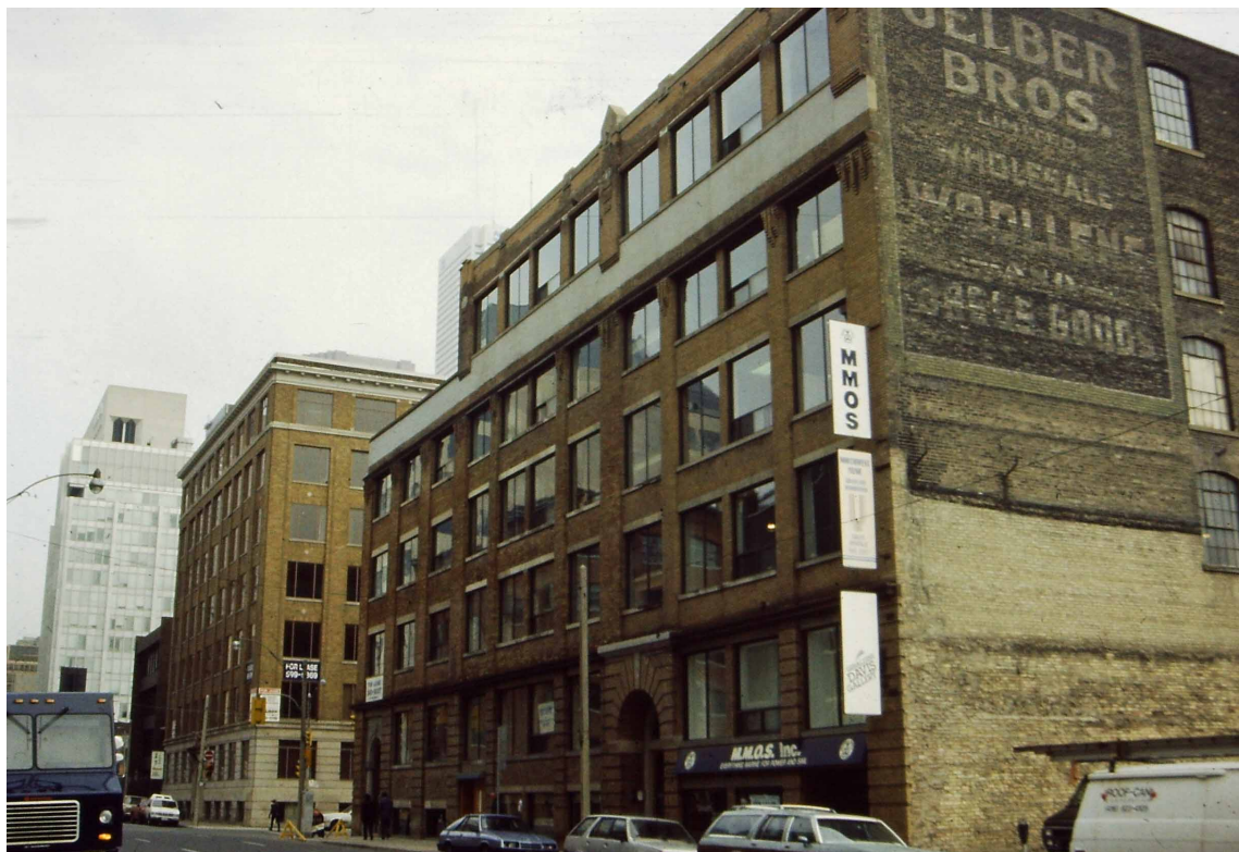
10. Richmond Street looking west with the Gelber Building on the right showing the "Gelber Brothers Limited" signage on the west façade, the five-and-a-half storey addition designed by Brown in 1923 and the original, four-and-a-half storey Gelber Building designed by Louis S Yolles in 1910 to the left. Across Duncan Street, to the left, is the New Textile Building, commissioned by the Gelbers in 1923-4 and designed by Brown. (Toronto Historical Board, April 1991)
