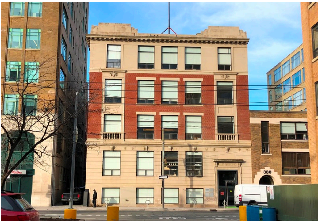
35. Ellis Building, 384 Adelaide Street West, flanked by the Balfour Building, 110 Spadina Avenue and 380 Adelaide Street West representing the architectural styles and scales of the immediate context of 355-359 Adelaide Street. (HP, 2020)
