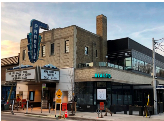
22. Benjamin Brown, Paradise Theatre, 1006 Bloor Street West (1937) with recent rehabilitation and additions including the Rialto restaurant initiated in 2014 (HP, 2020)
