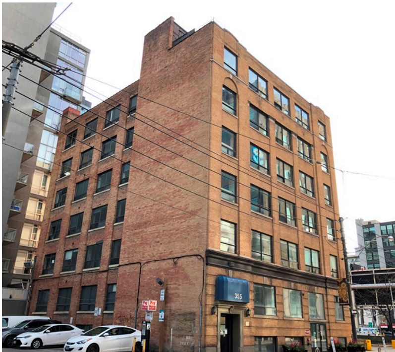
33. Principal (north) and side (east) elevations at 355-359 Adelaide Street West (HP, 2020)
