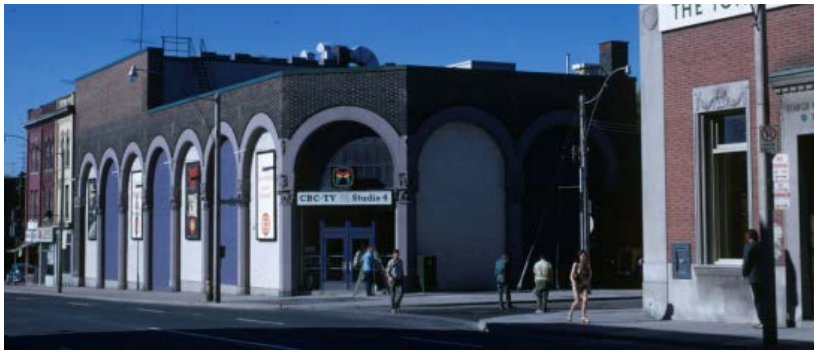
10. 1971 archival photograph showing the closed in arcade during the building's time as a film production studio for the CBC. The cast stone cornice and other decorative details are missing by this point. At left is the adjacent commercial row at 1130-1134 Yonge Street. (CoT Archives)
