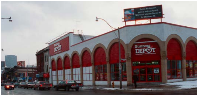
11. 1990s archival photograph showing the building under ownership by The Business Depot, later Staples Canada. At this time, several of the arcade openings on the east and north elevations were re-glazed. (CoT Archives)
