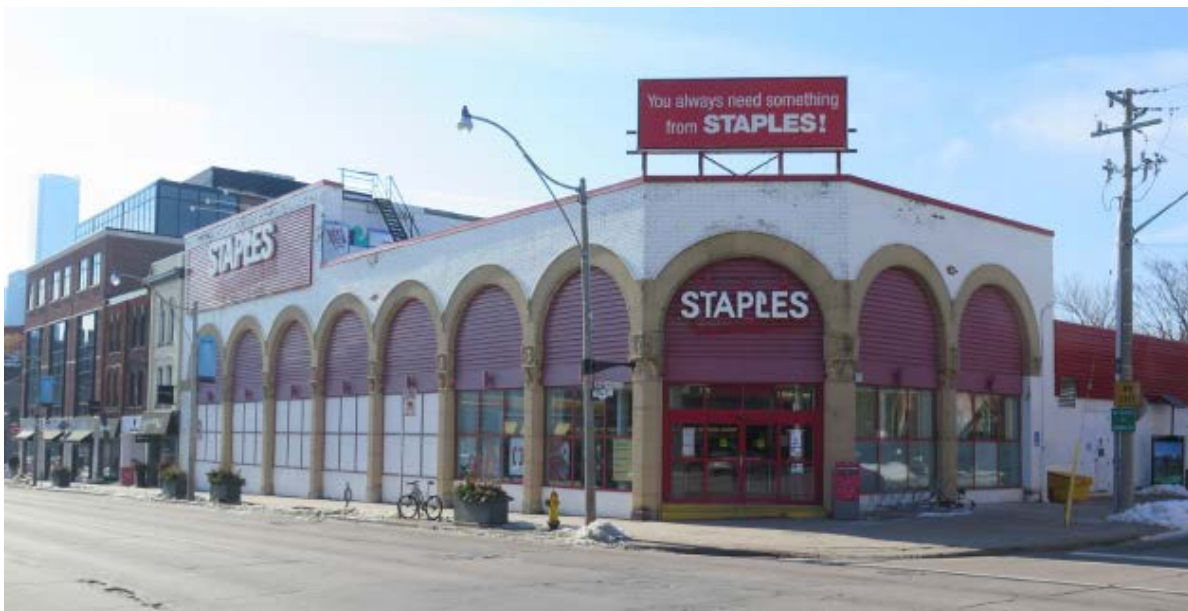
East and north elevations of 1140 Yonge Street at the corner of Marlborough Avenue (ERA, 2020)
