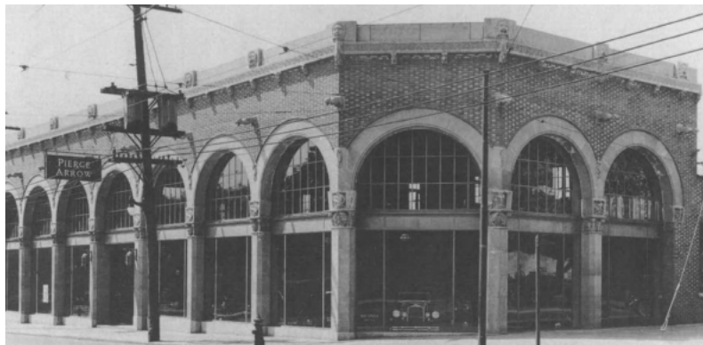
9. 1930 archival photograph of the recently completed Pierce-Arrow showroom. Note the projecting gargoyles in the arcade spandrels, now lost. (CoT Archives)
