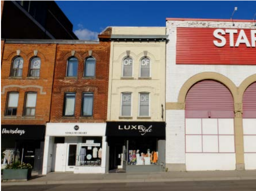
East elevation of the main street commercial row at 1130-1134 Yonge Street with part of the adjacent property at 1140 Yonge visible at right (ERA, 2020)
