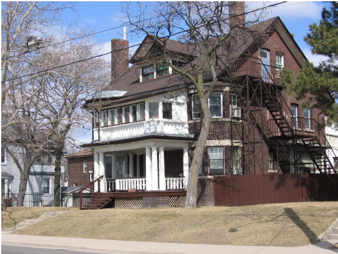
17. View of the principal west and side, south elevations and the setting of 537 Broadview Avenue (HP, 2009)
