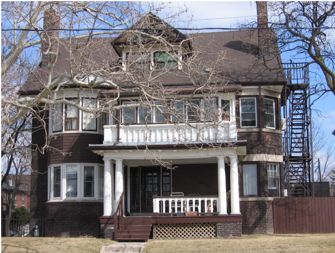
14. 537 Broadview Avenue: principal, west, elevation (HP, 2009)
