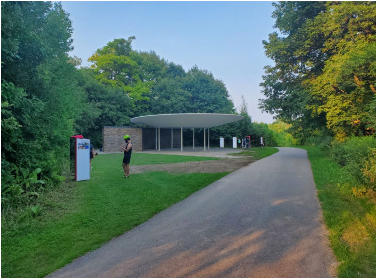
Figure 34. View of the South Humber Park Pavilion walking east on the Humber River Recreational Trail (Heritage Planning, 2021)
