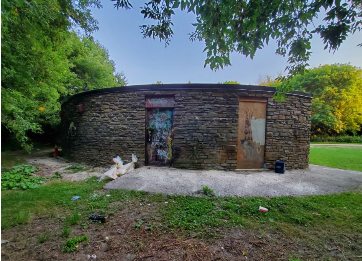
Figure 19. Detail of the men's washroom entrance in the rear (north) elevation (Heritage Planning, 2021)
