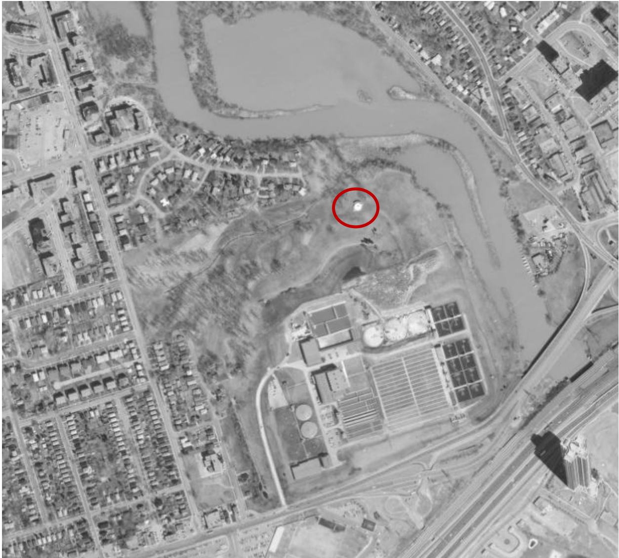
Figure 6. 1978 Aerial photograph showing the completed South Humber Park Pavilion and the Humber Wastewater Treatment Plant (City of Toronto)
