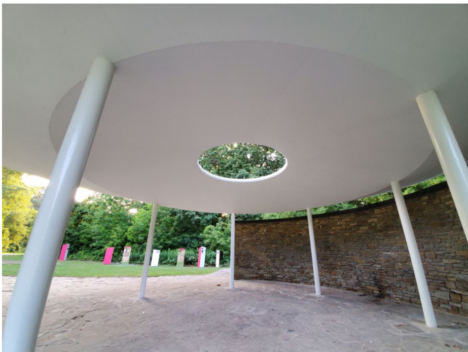
85 Stephen Drive, detail of the oculus in the canopy of the shelter structure (Heritage Planning, 2021)
