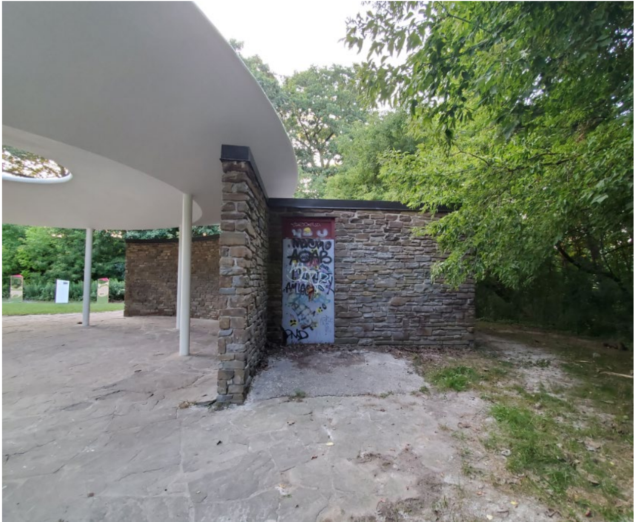
Figure 18. Detail of the women's washroom entrance in the side (east) wall (Heritage Planning, 2021)
