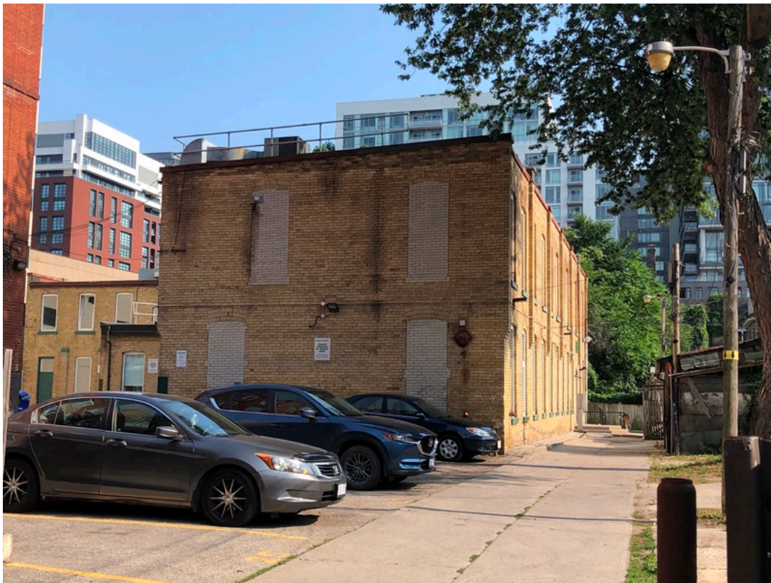
16. Original approach to and view of the E. C. Walker & Sons Ltd. factory from the laneway from Richmond Street West, with its principal elevation facing west towards Bathurst Street (HP, 2021)
