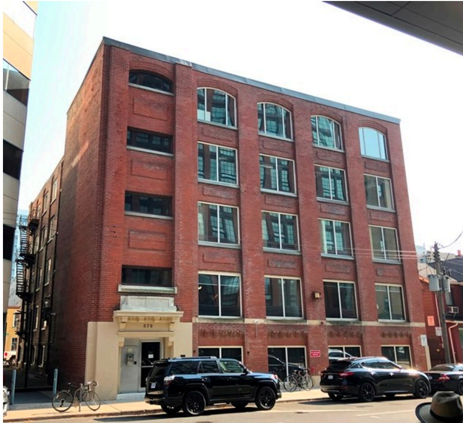
Independent Cloak Co., 579 Richmond Street West, principal (north) elevation (HP, 2021)
