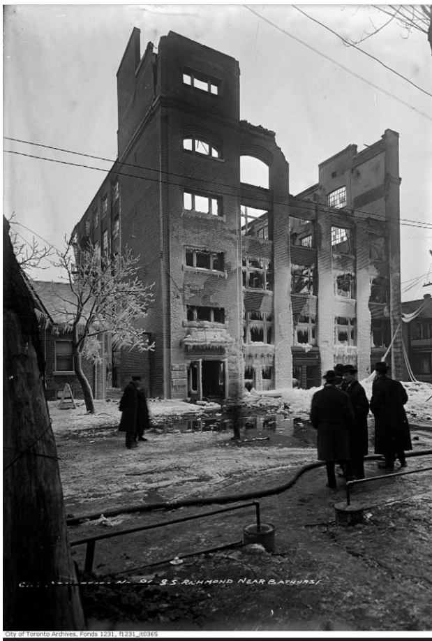
35. James Salmon photograph, "Fire on the South Side of Richmond Street", date February 6, 1914, showing the Independent Cloak Co. building after the fire (City of Toronto Archives, Fonds 1231, f1231, it0365)
