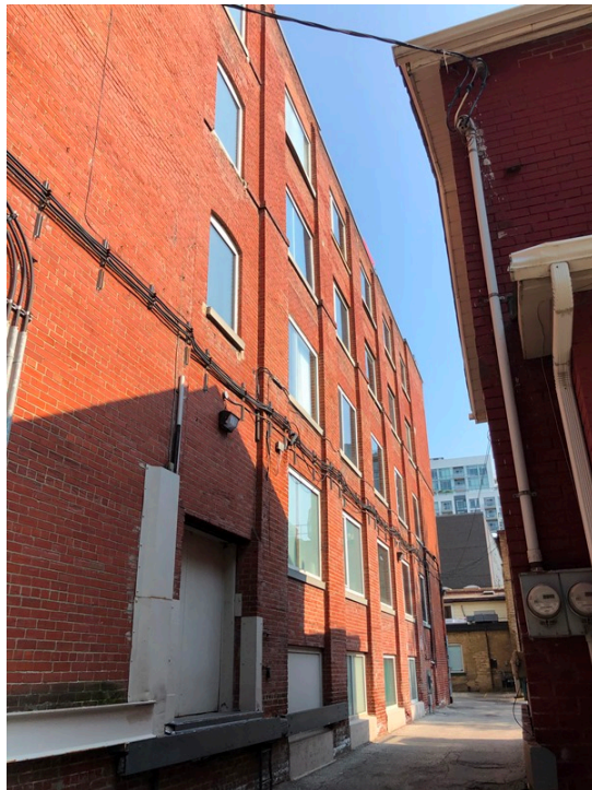
39. Side, west elevation, Independent Cloak Co., looking south, past the loading door along the laneway to E. C. Walker & Sons factory yard (HP, 2021)
