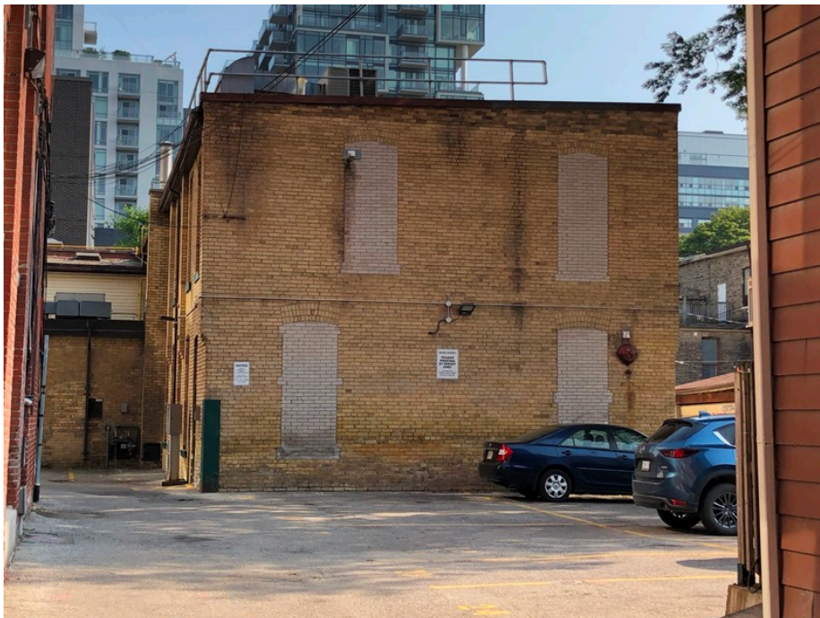
20. Side elevation facing north, E. C. Walker & Sons Ltd., as viewed from the laneway on the west side of 579 Richmond Street West. (HP, 2021)
