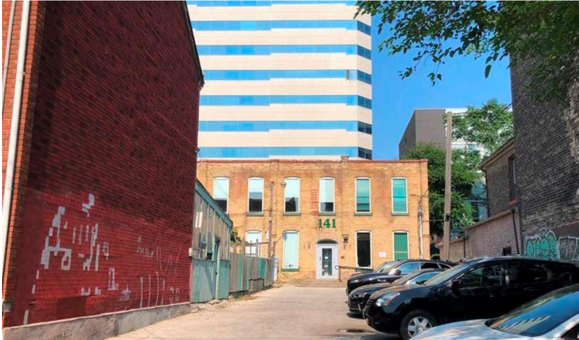
15. View of the E. C. Walker & Sons Ltd. factory, 141 Bathurst Street, from Bathurst Street with its principal entrance at the south end of its west elevation (HP, 2021)
