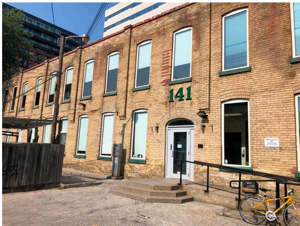
E. C. Walker & Sons, Ltd., 141 Bathurst Street, principal (west) façade (Heritage Planning [HP], 2021)
