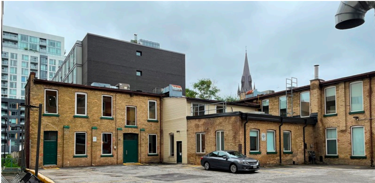
22. Rear, east side, E. C. Walker & Sons Ltd., showing the north elevation of the later addition, the two-storey infill, clad in aluminum siding, the original single storey wing and the east elevation of the main block (HP, 2021)
