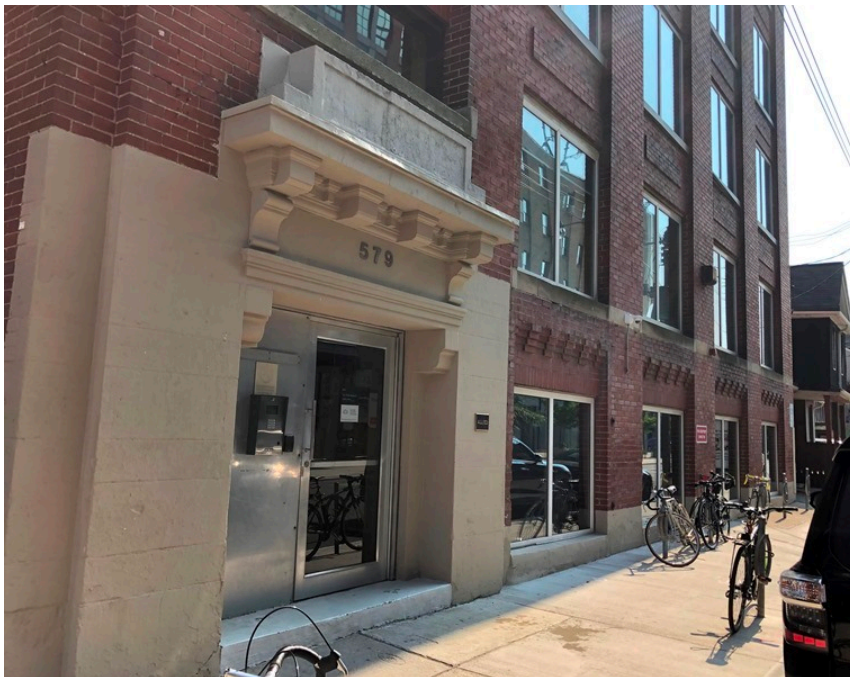
37. Principal, entry with art stone door case, north elevation, Independent Cloak Co. (HP, 2021)
