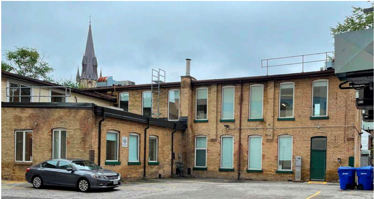
21. Rear elevation facing north, E. C. Walker & Sons Ltd., showing the east elevation of the main block and the single storey wing. The spire of St. Mary's church is seen in the distance (HP, 2021)
