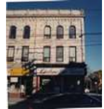
Figure 1: 1996 picture. South elevation
