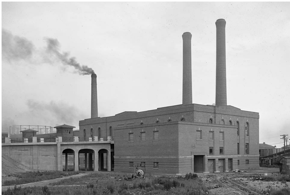
Figure 1: Image of the Wellington Destructor in 1925
