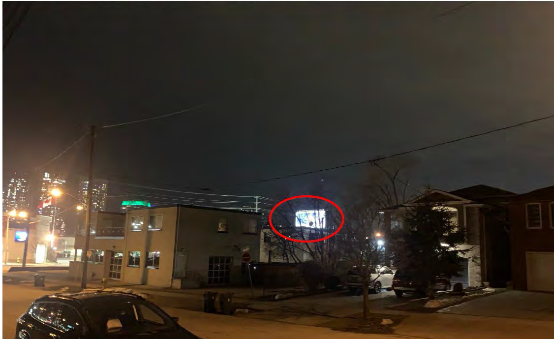
Existing Sign from nearest home on High Street
