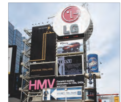
Media Tower installed on building
