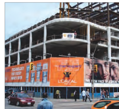
Signage applied to temporary hoarding
