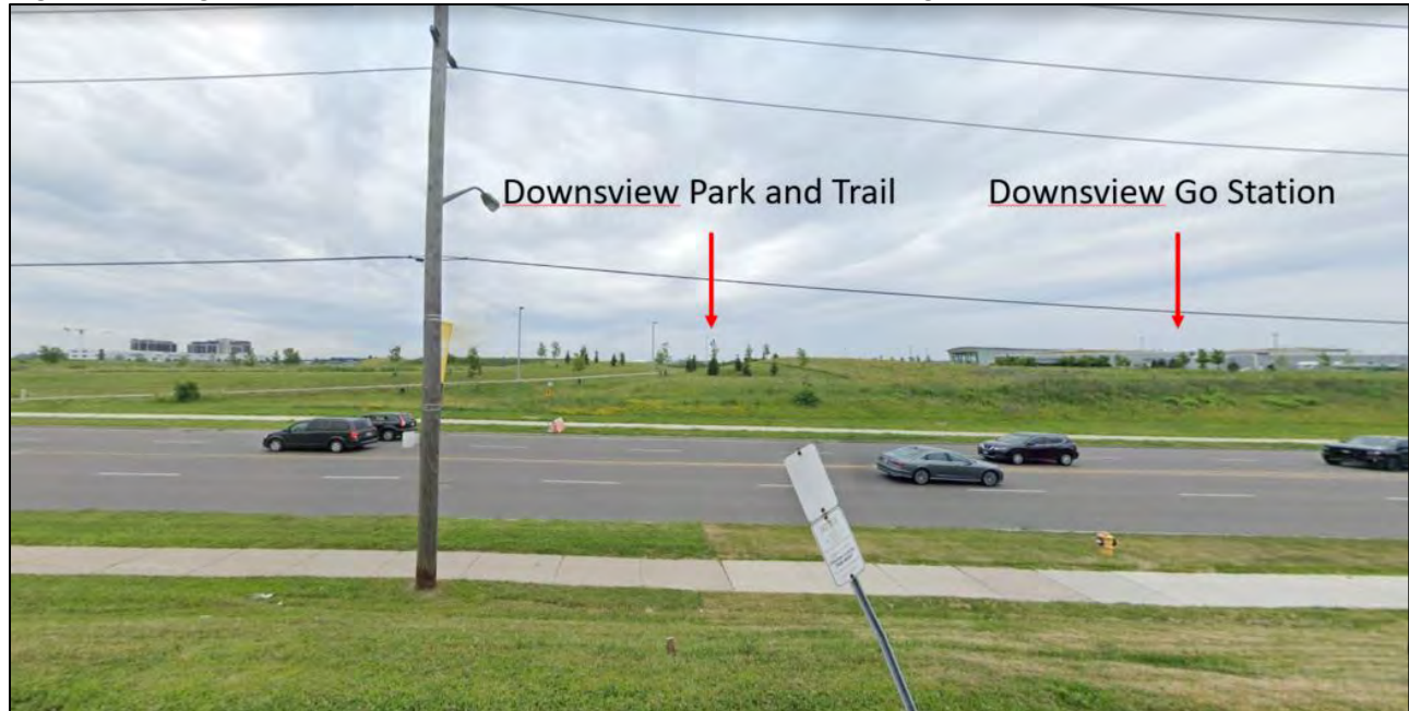
Figure 8- Google Street View – 3848-3998 Chesswood Drive looking south:
