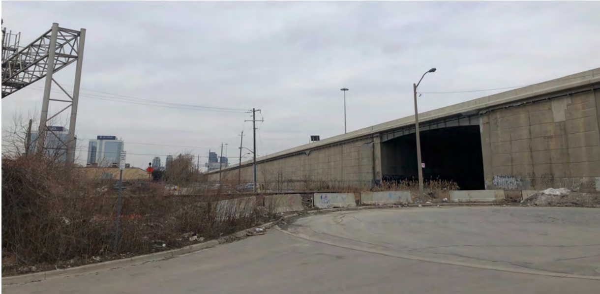
Looking northeast to subject site, at CP Rail corridor and Highway 427 overpass
