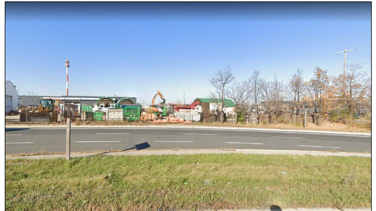
Figure 4: View From Highway 409 toward The Premises
