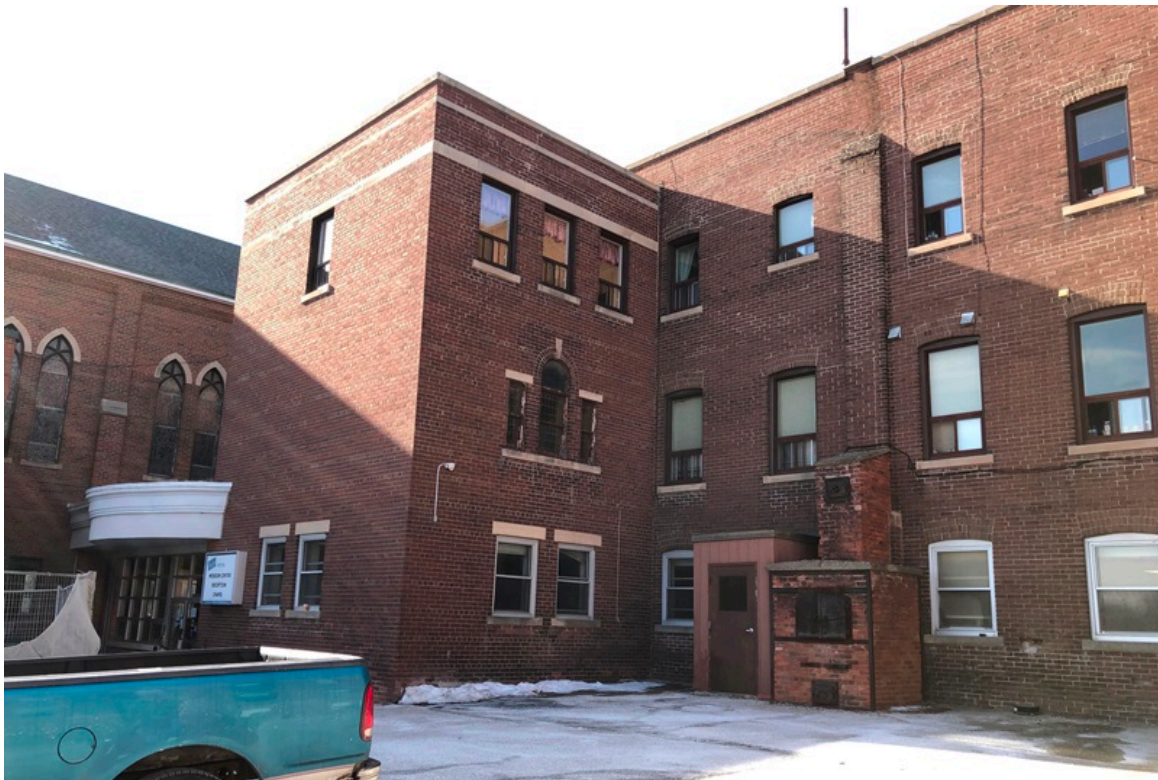
28. Photograph showing the 1933 extension of the original chapel with the Palladian window, (centre) the south elevation of the 1923-4 seminary (right) and the 1958-9 chapel with later, 2005-6 entrance (left)
