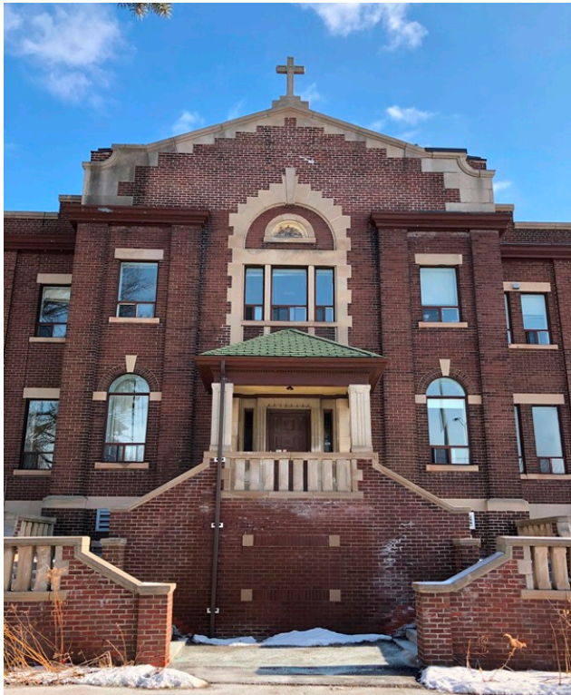
16. North elevation showing the central frontispiece with the staircase and later porch (1939)
