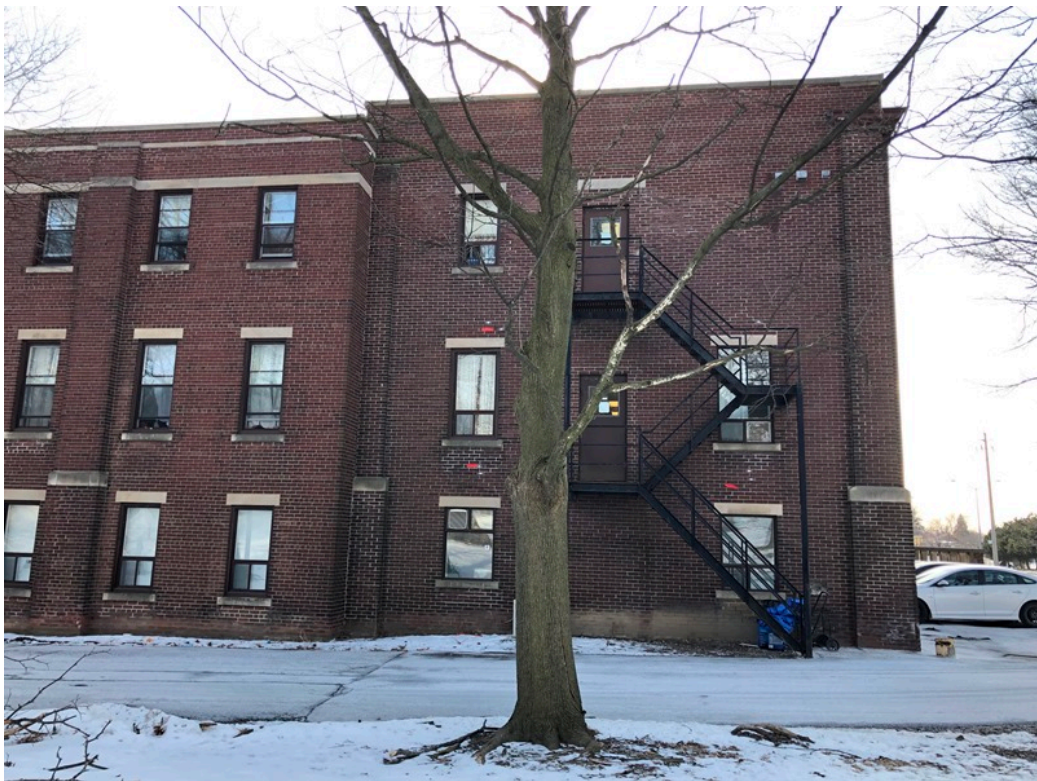
25. Photograph showing the east elevation with the original 1923-4 and to the left the addition in 1933
