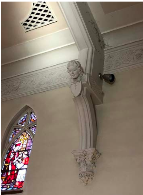
49. Chancel area corbel bracket with angel and Corinthian capital typical of the High Gothic period (1220-1260), frieze with grapes and vines and ceiling return air screen
