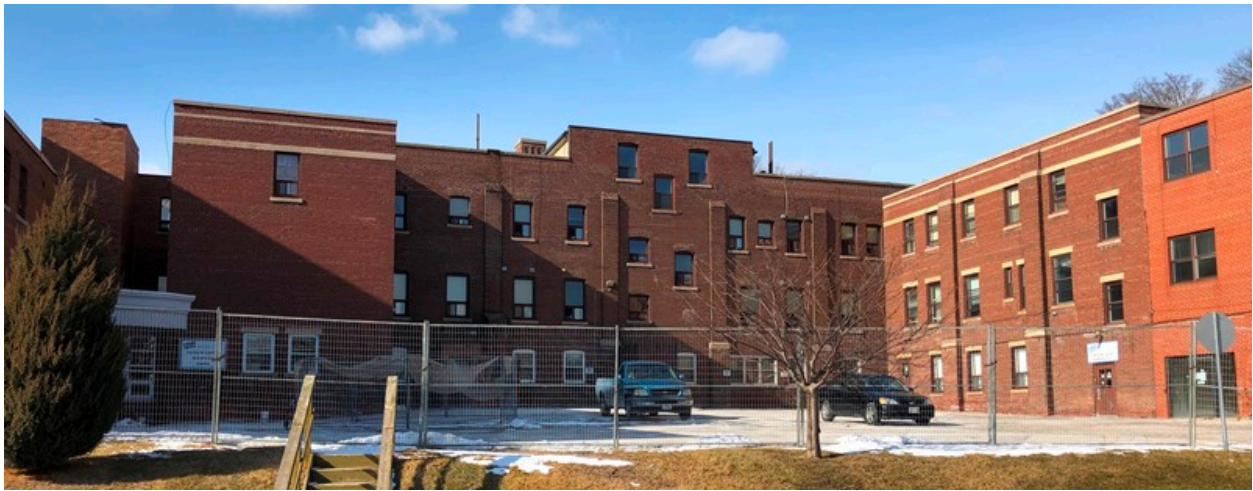
27. South elevation of the original 1923-4 Seminary, (centre) with 1933 extensions (left and right) and 1956 extension (far right)
