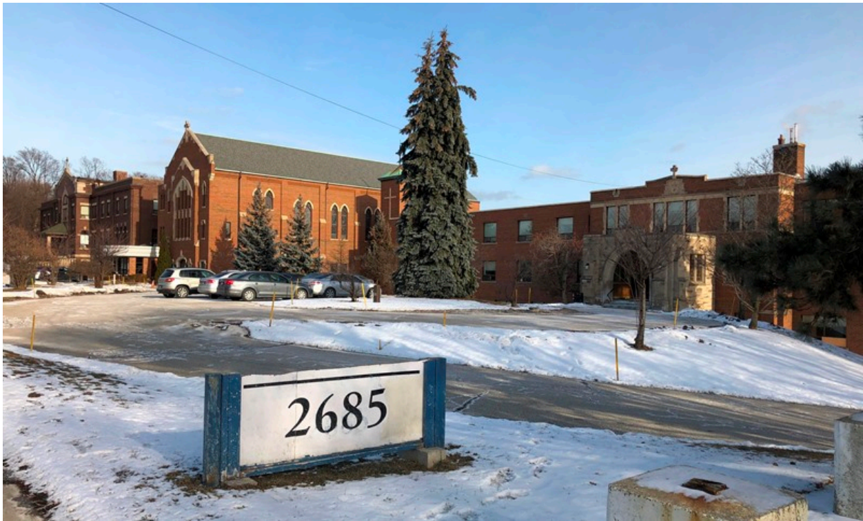
35. View of the Scarborough Foreign Mission Society complex with the 1958-9 additions, with forecourt and the slope in the landscape towards the residential wing
