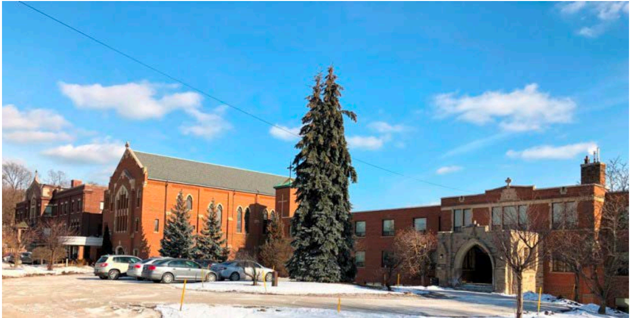
Photograph of the Scarboro Foreign Mission Society, 2685 Kingston Road, looking east from Kingston Road (Heritage Planning, 2021)
