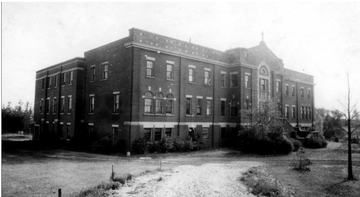
24. Photograph of the Seminary building taken after the 1933 addition but prior to the addition of the 1939 porch. Note the stone square patterning on the parapet, removed with later repairs (Scarboro Foreign Mission Society, "1918-2018 Moments in History")
