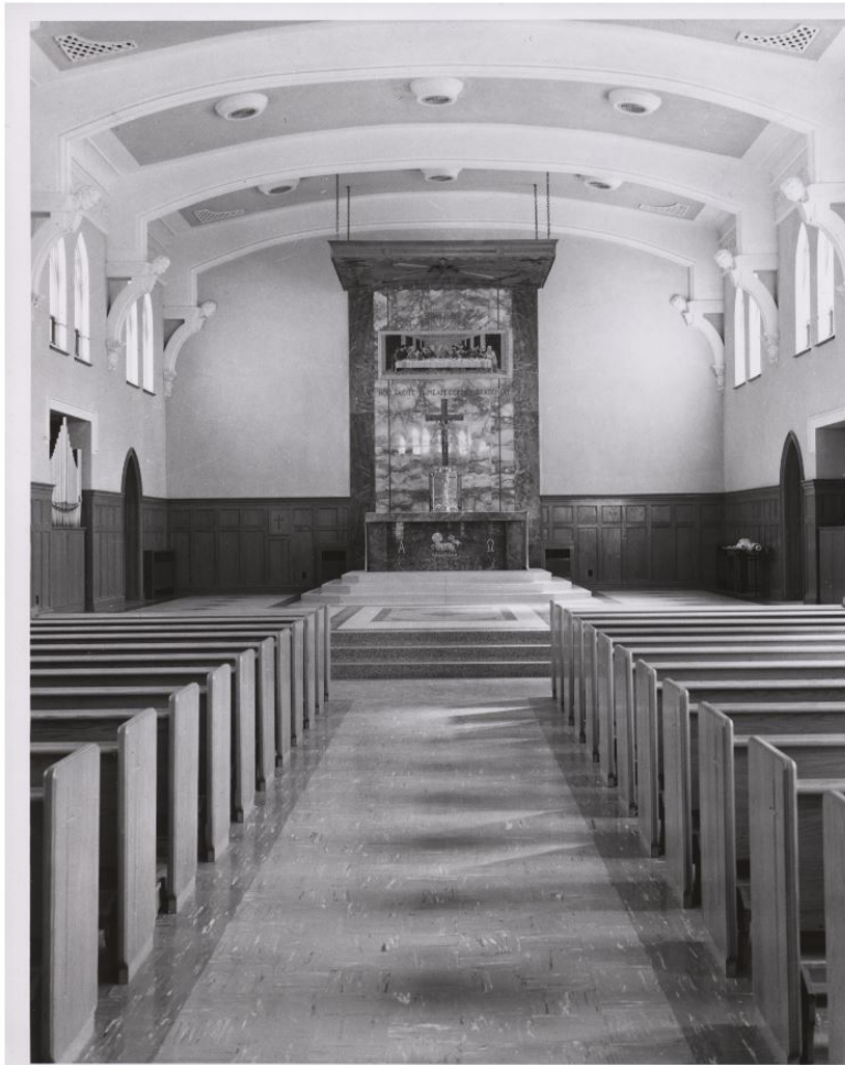
45. Photograph taken in 1959 of the chapel interior after completion. (SFMSA)
