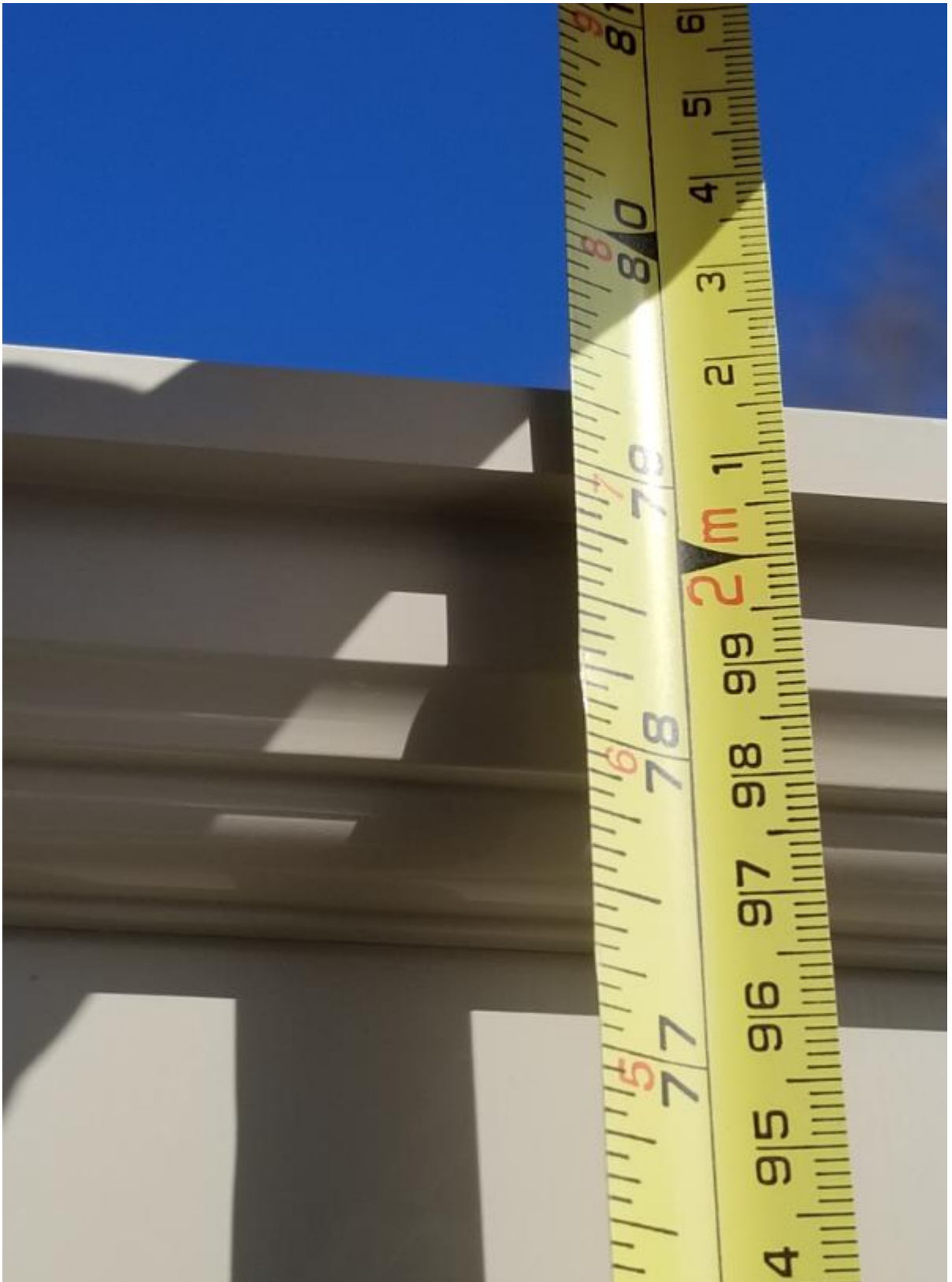
Appendix #3 - Height of existing PVC composite fence at 25 Conference Blvd rear yard.
