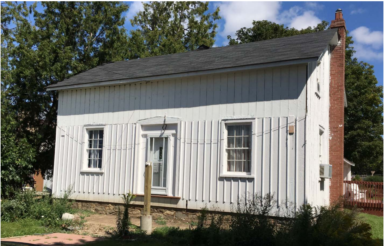
13. West Elevation of the George L'Amoreaux farm house (HP, 2017)
