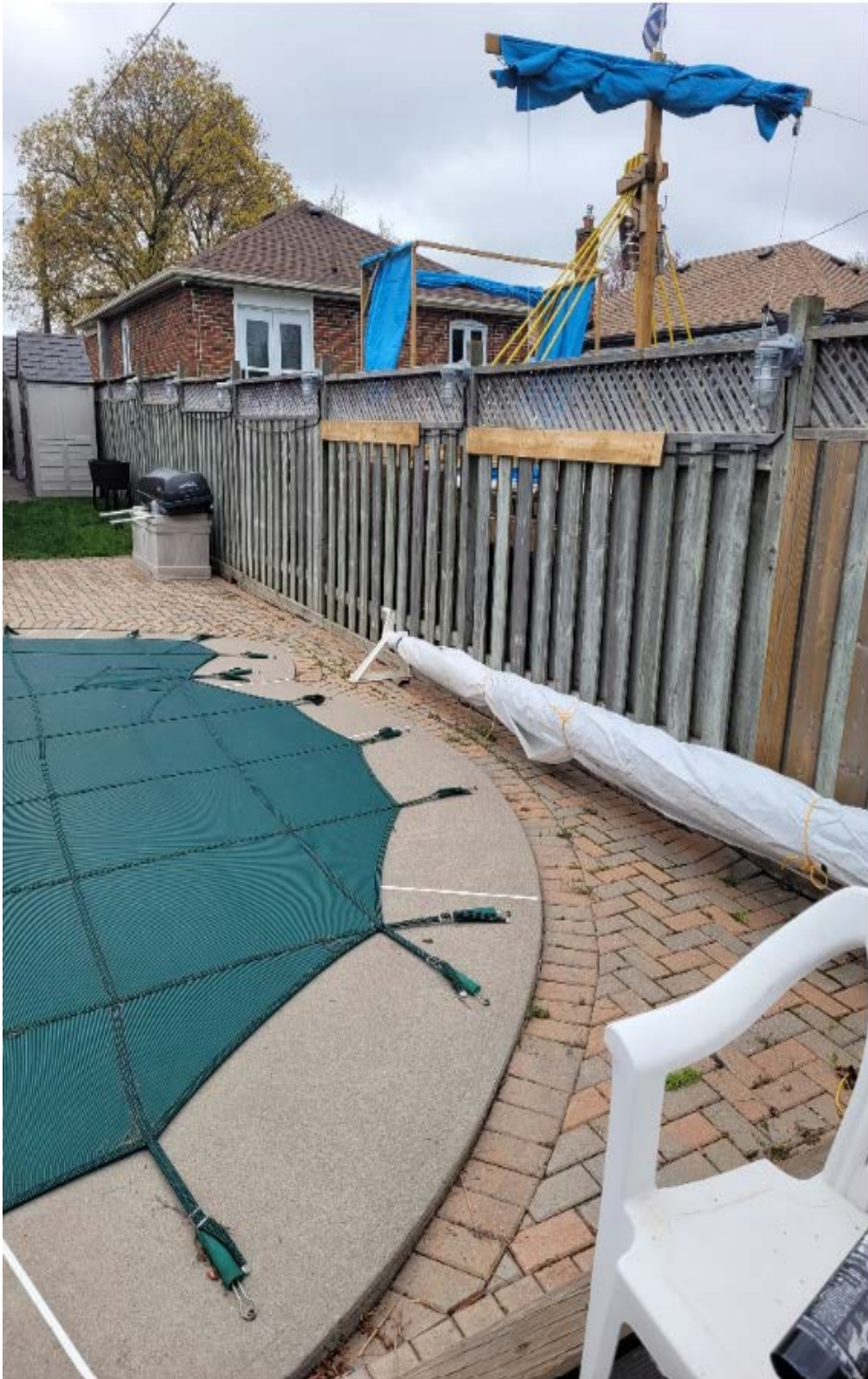
Elevation photo taken of 28 Ilfracombe rear yard.
