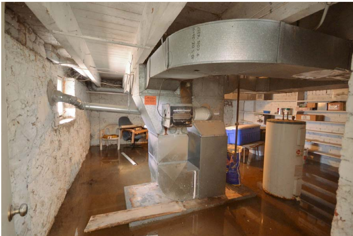
Fig. 67 Two-roomed cellar, looking west and showing outer walls of rubble stone and a brick partition wall running east to west. Note water pooled on the cellar floor.
