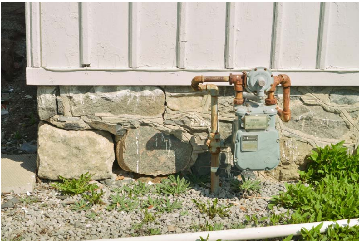
Fig. 41 South elevation rubble stone foundation wall at farmhouse's southwest corner, showing some mortar joints missing
