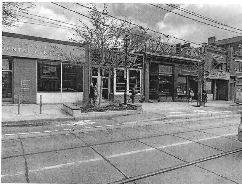
233 Roncesvalles Avenue – Front (West) Elevation
