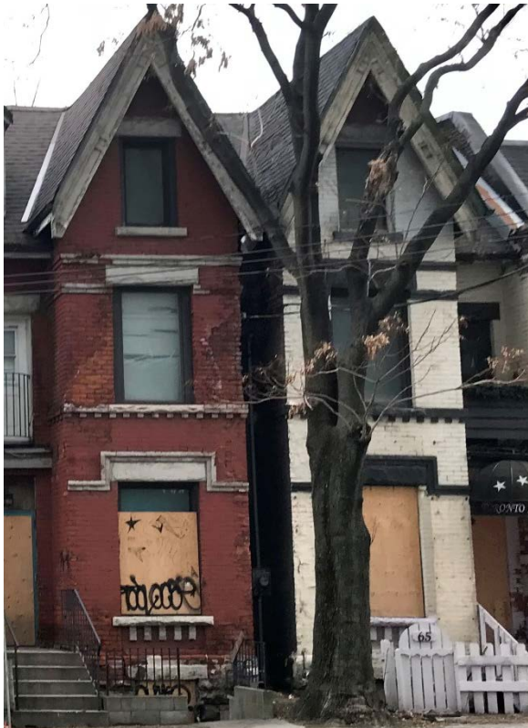
Figure 7. View of 63-65 Elm Street showing the 2.5-story square bay surmounted by a steep-pitched gable, and the decorative stonework above the first and second floor window openings. (Heritage Planning, 2021)
