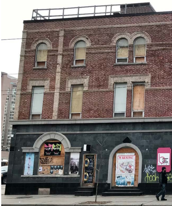
Figure 6. Detail of the round and flat-hooded window openings on the east elevation, including the Palladian windows at the ground level. (Heritage Planning, 2021)
