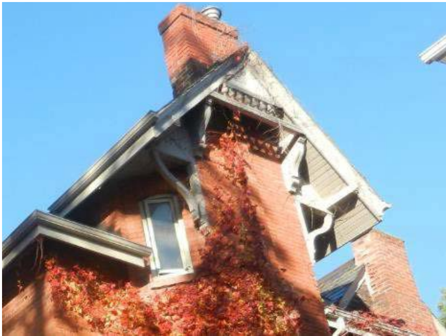
Figure 4. View of the chimney on the east elevation and gable with its deep brow, decorative wooden bargeboard and curved brackets (AREA, 2020)
