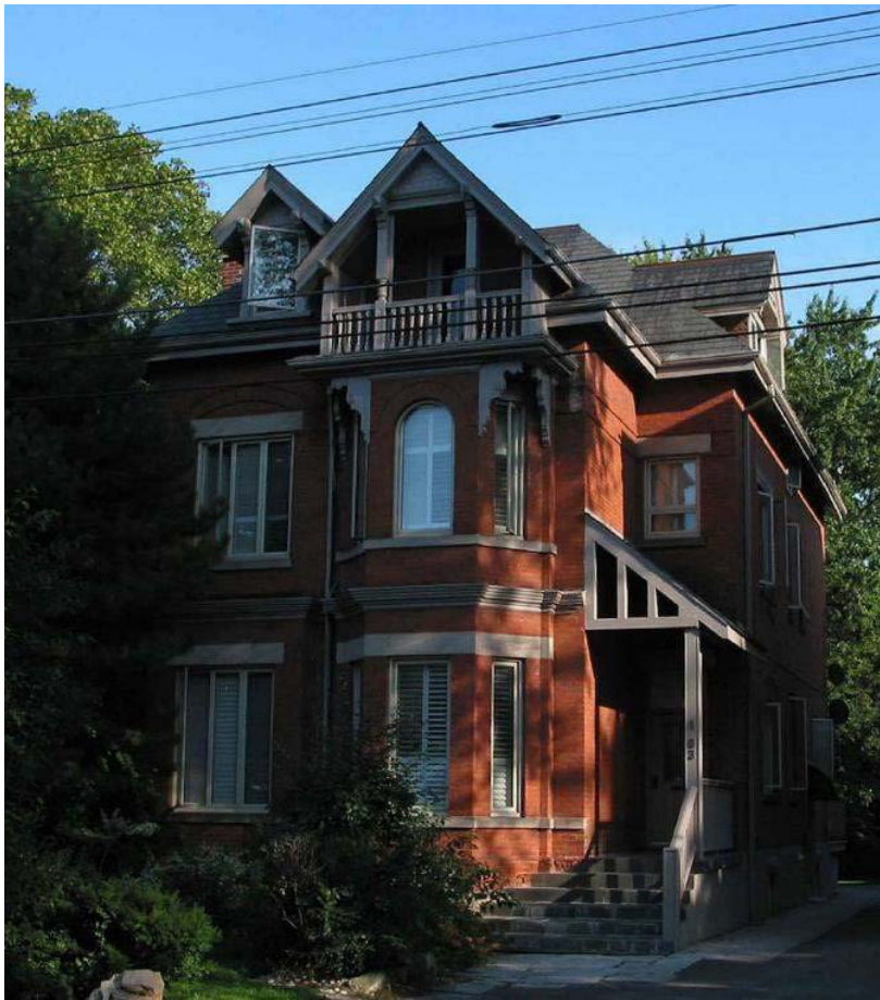
Figure 2. View of the principal (north) elevation (AREA, 2020)
