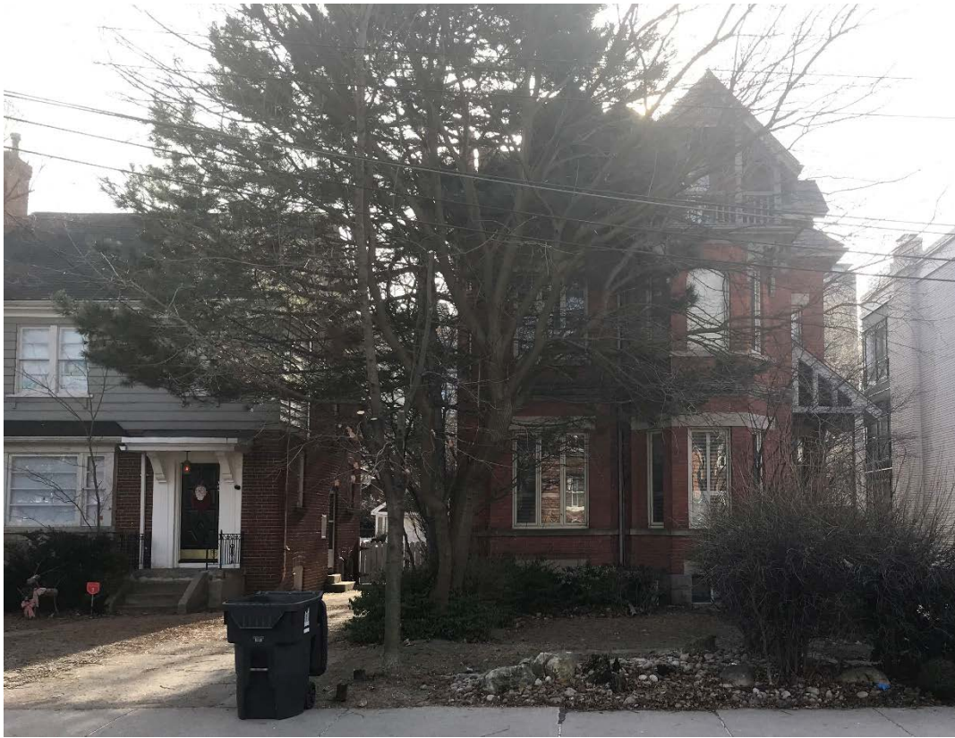
Figure 6. View of the properties at 101 and 103 Heath Street West, both of which are subject to the current development application (Heritage Planning, 2020)
