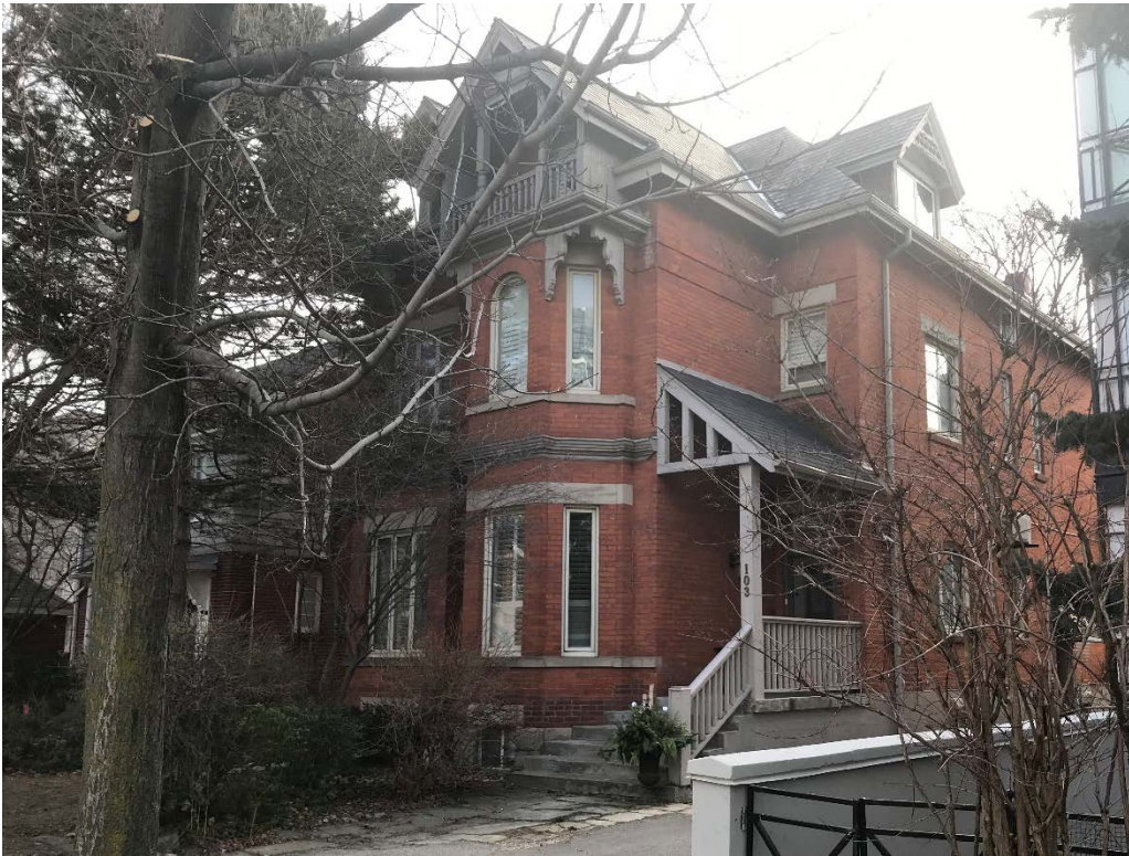
View of the principal (north) elevation and west elevation (Heritage Planning, 2020)
