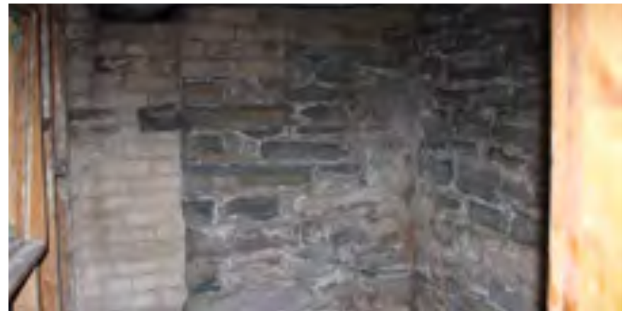
Typical rubble stone foundation wall
