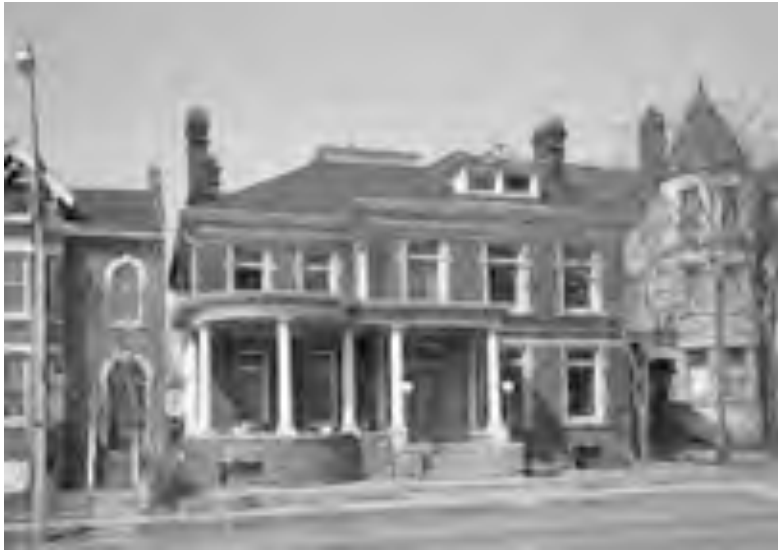
1970s - the house prior to the application of an exterior stucco
