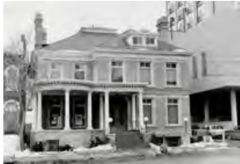
1980s - the house after the application of the exterior stucco
