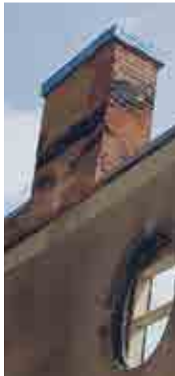
Remaining north masonry stack (Source: GBCA, 2020)
