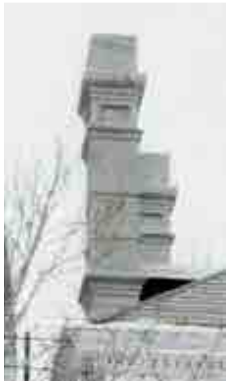
Decorative south masonry chimneys, c.1981 (Source: Toronto Public Library)
