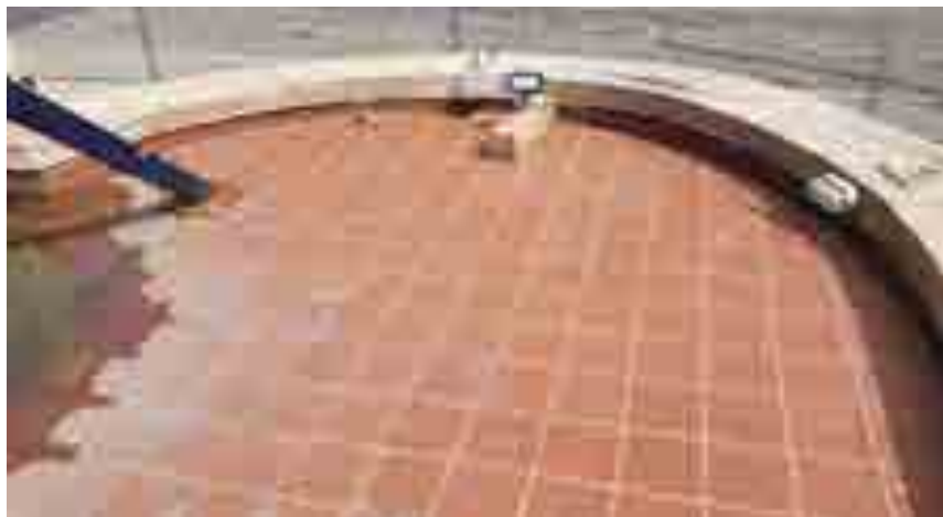
Image showing non-original ceramic tile flooring to be removed (Source: GBCA, 2020)
