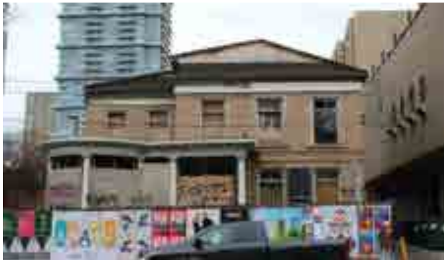
Image showing 314 Jarvis condition after the 2016 fire, the original roof was destroyed during the fire and replaced with a temporary roof structure (Source: GBCA, 2019).
