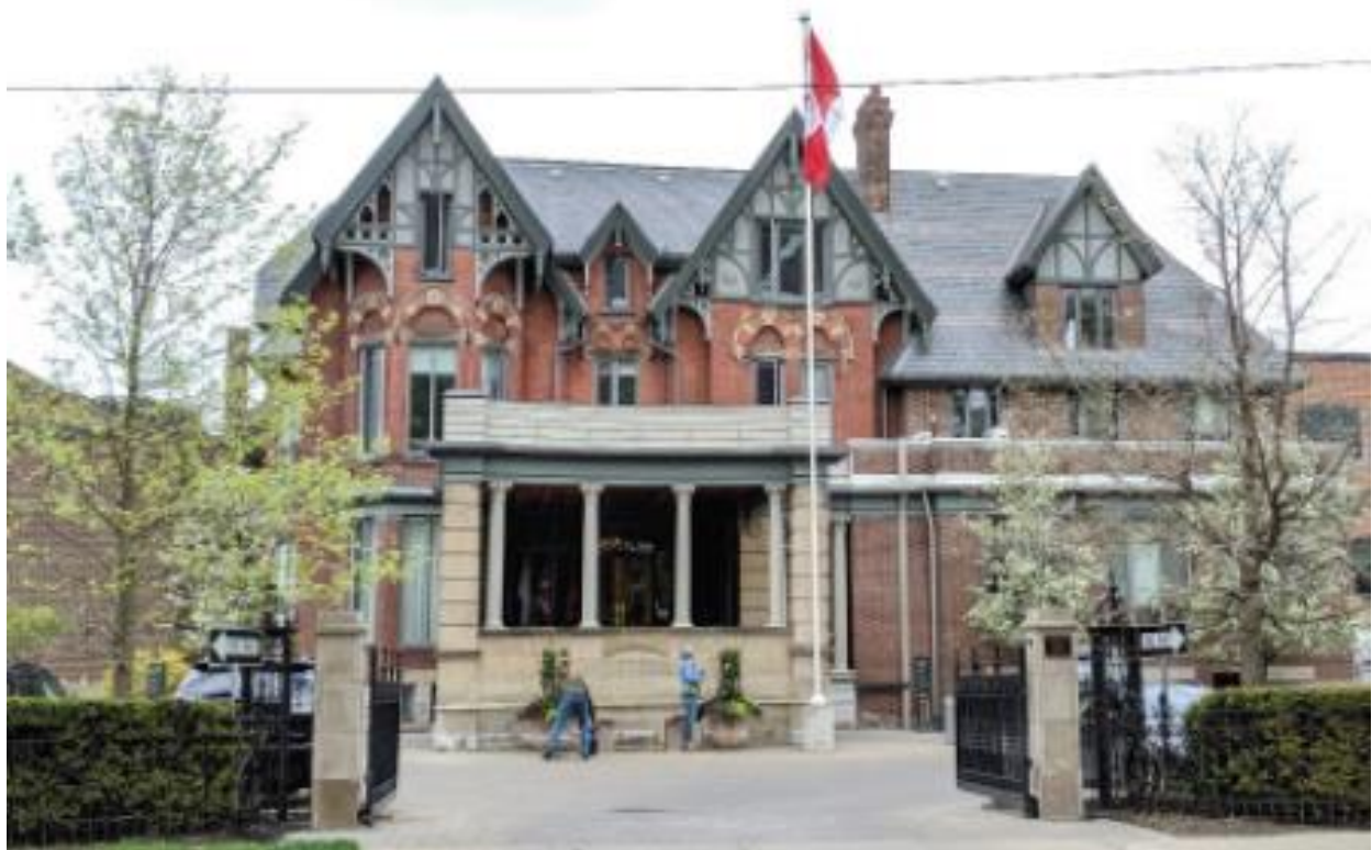
View of primary (south-facing) elevation of "Hollydene" (1879), with the 1930 Senior Common Room addition to the east, at 10 Elm Avenue
