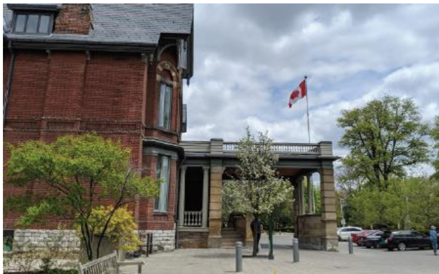
View of secondary (west) elevation of "Hollydene" and its porte cochere at 10 Elm Avenue
