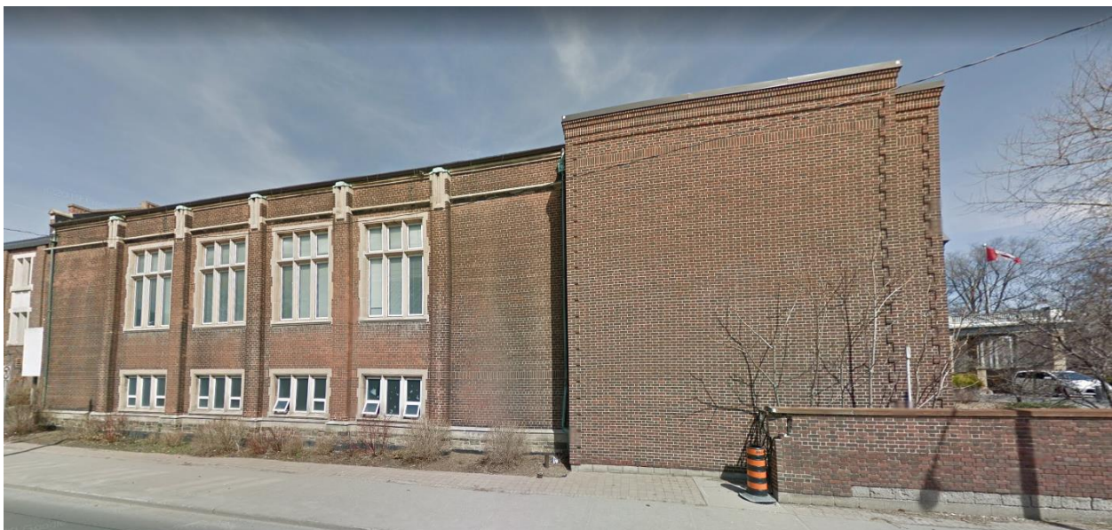
View of the west elevation of the 1924 Gymnasium and Classroom addition and 1978 addition at 10 Elm Avenue (2014 image shown, prior to tree growth along the side of the building)
