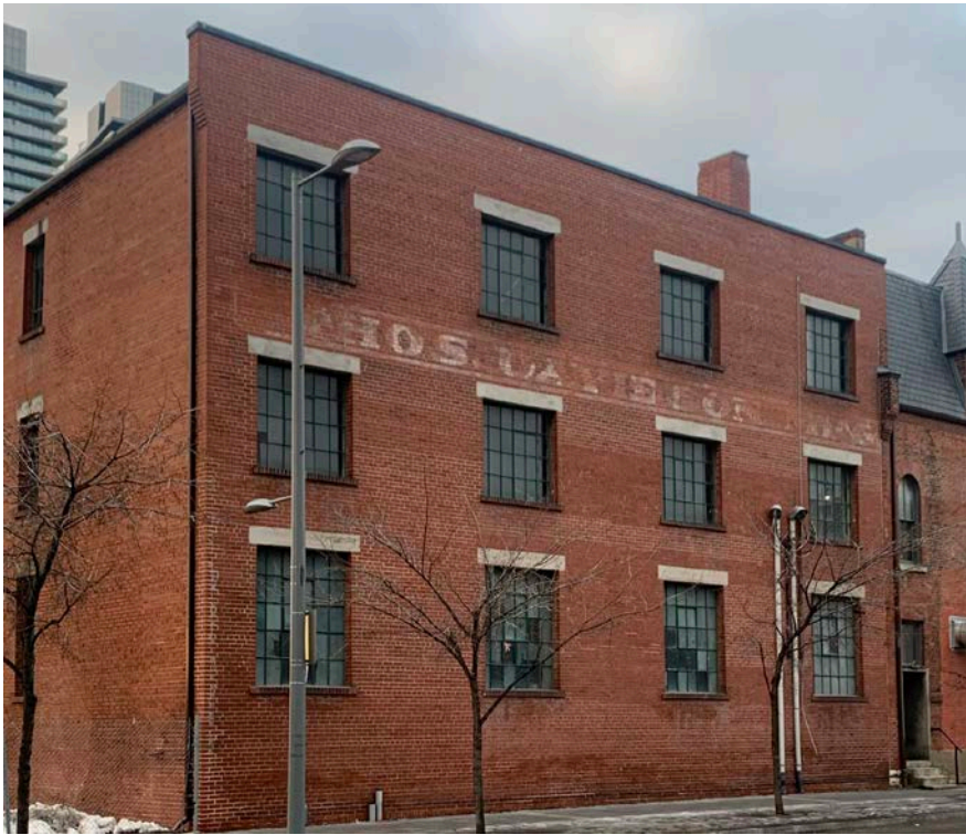
29. 425 Cherry Street, north façade, warehouse addition (Heritage Planning, 2021)
