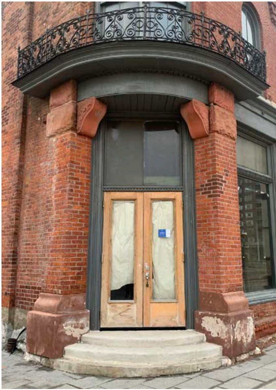
31. 425 Cherry Street, northwest façade, detail of corner entrance (Heritage Planning, 2021)
