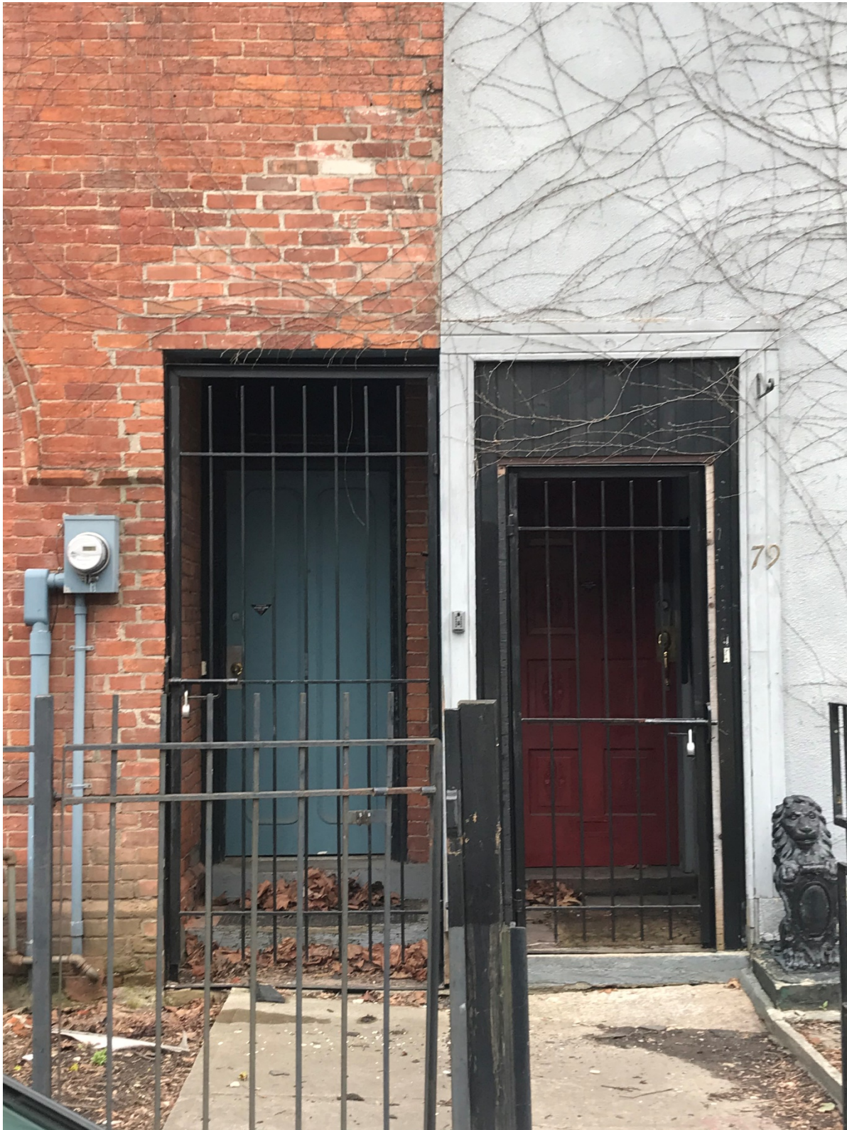
Image 9. Current photograph showing the main entrances to the subject properties at 79 and 81 Granby Street which were altered at different times from their original design, which included a shared, round-arched entryway. (Heritage Planning, 2021)
