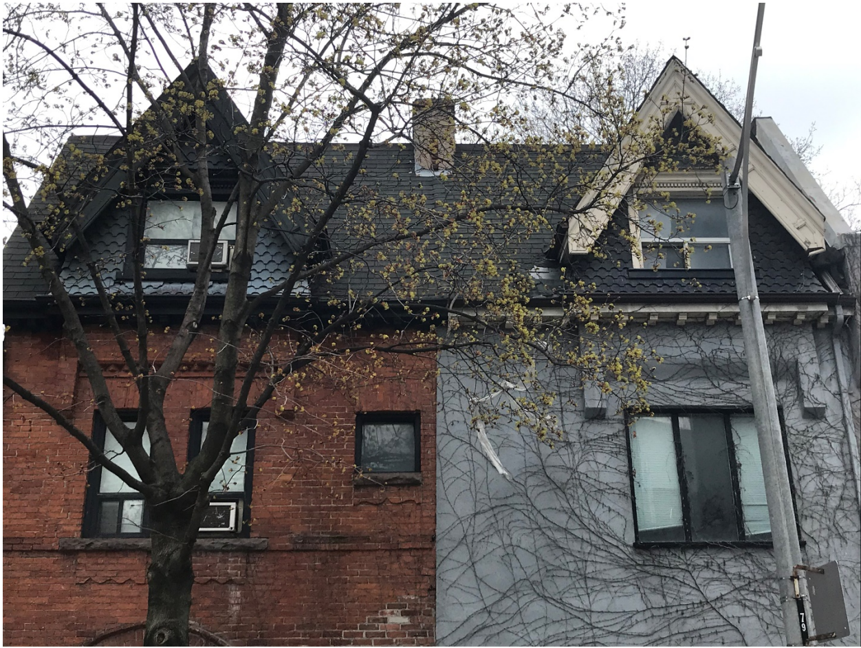
Image 3. Current photograph showing the second- and attic- storeys of the subject properties. While the openings at the second-storey level have been altered at 79 Granby, the attic storey form, arrangement, style and materials are original. (Heritage Planning, 2021)
