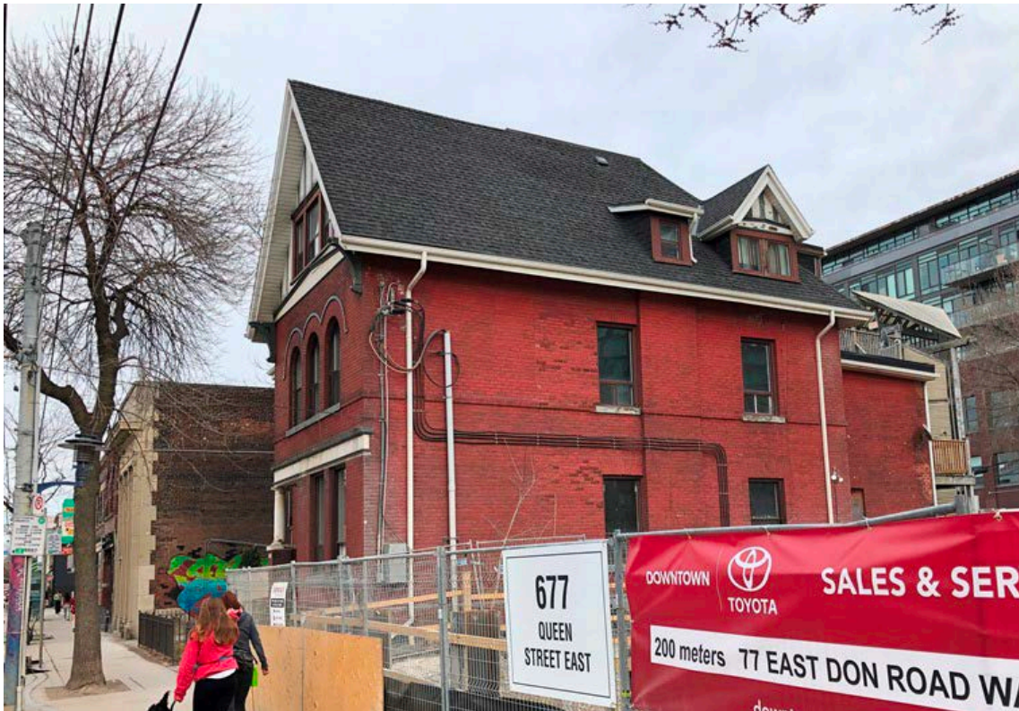
13. 685 Queen Street East: photograph showing the side, west elevation and roof top dormer windows. (HP, 2021)
