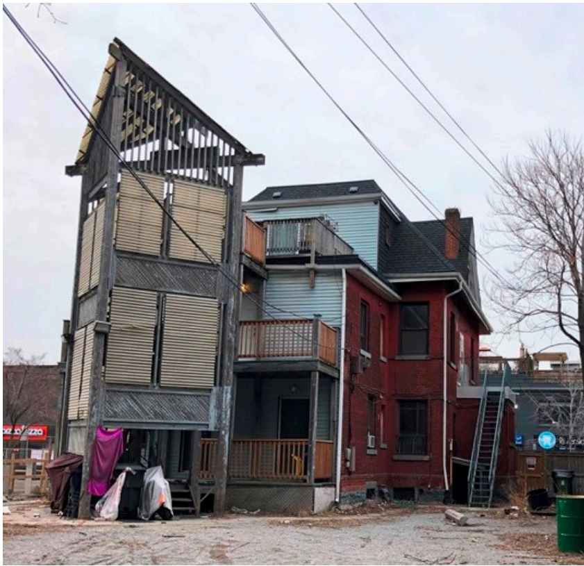
11. 685 Queen Street East, south and east elevations with rear wing: photograph showing the south side of the house with the rear, lower wing and the modern addition of a screened fire escape. (HP, 2021)
