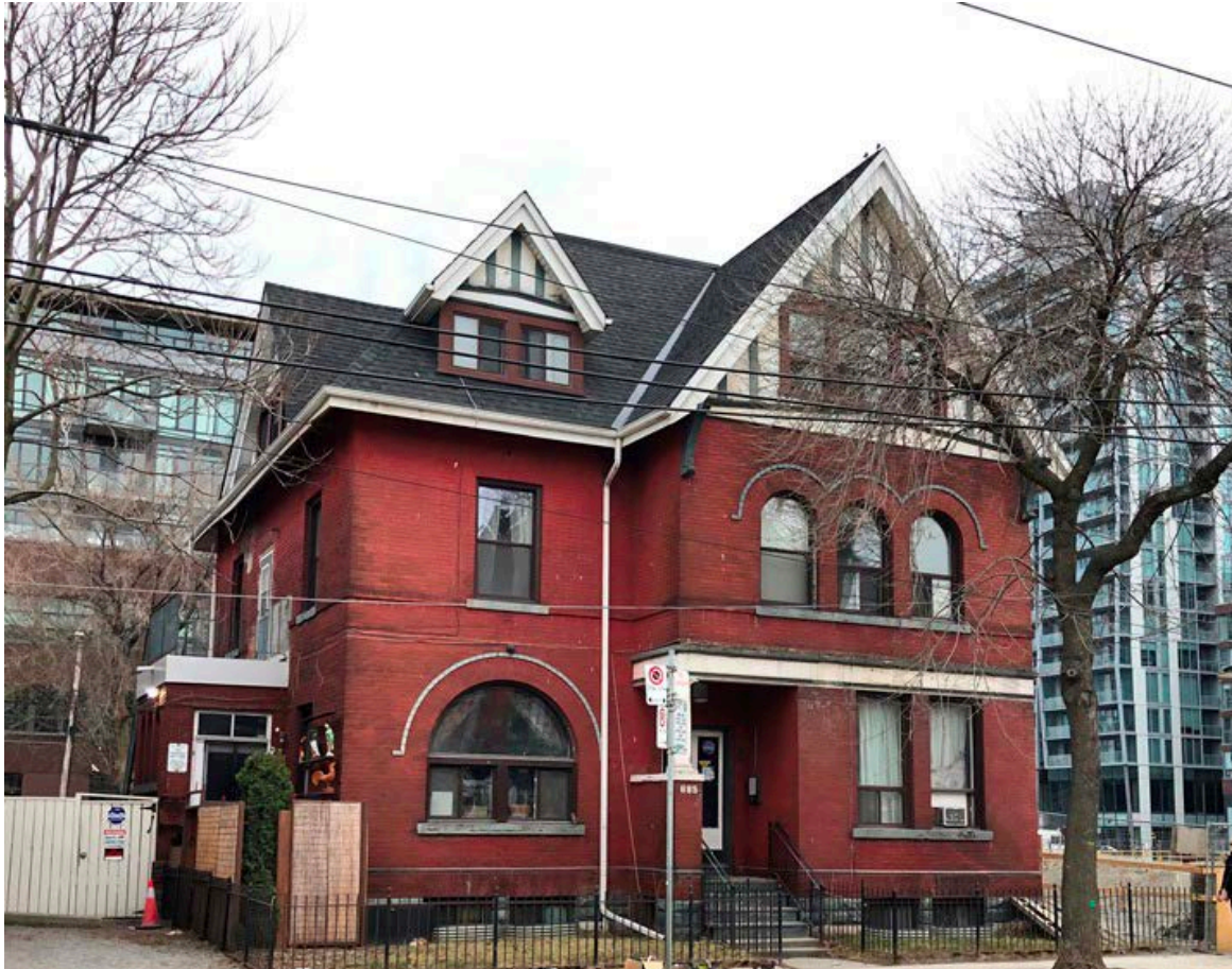
The Dr. John B. Fraser Office and Residence, 685 Queen Street East (Heritage Planning, 2021)
