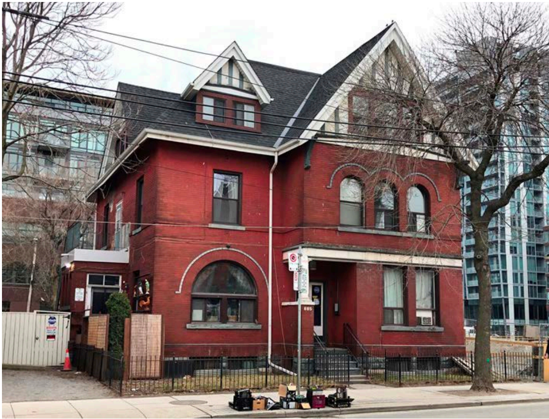
7. 685 Queen Street East: showing the principal, north, elevation and the east, side, elevation of the Dr. John B. Fraser house. (HP, 2021)
