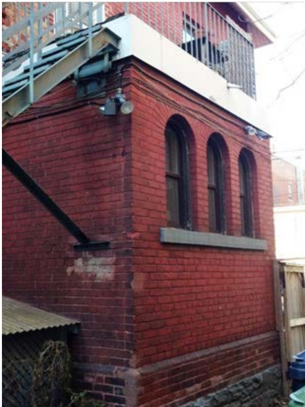
10. 685 Queen Street East, medical office entry porch, east elevation: Photograph showing the triple arched windows and continuous sill of the side entry porch and the brick details at the base. (HP, 2015)
