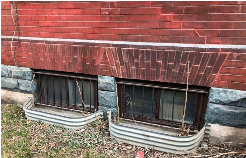
15. 685 Queen Street East, North Elevation, Detail of the stone foundation and the brick work: Photograph showing the details of the stone foundation and the brickwork on the principal, north elevation. Note the careful patterning and mortar joints of the paired basement windows (HP, 2021)
