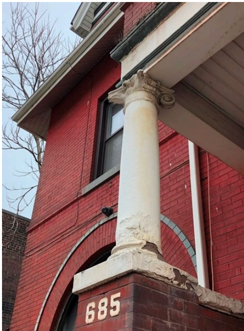
8. 685 Queen Street East: Photograph showing the single, composite column supporting the projecting bay above the front entry loggia. (HP, 2021)
