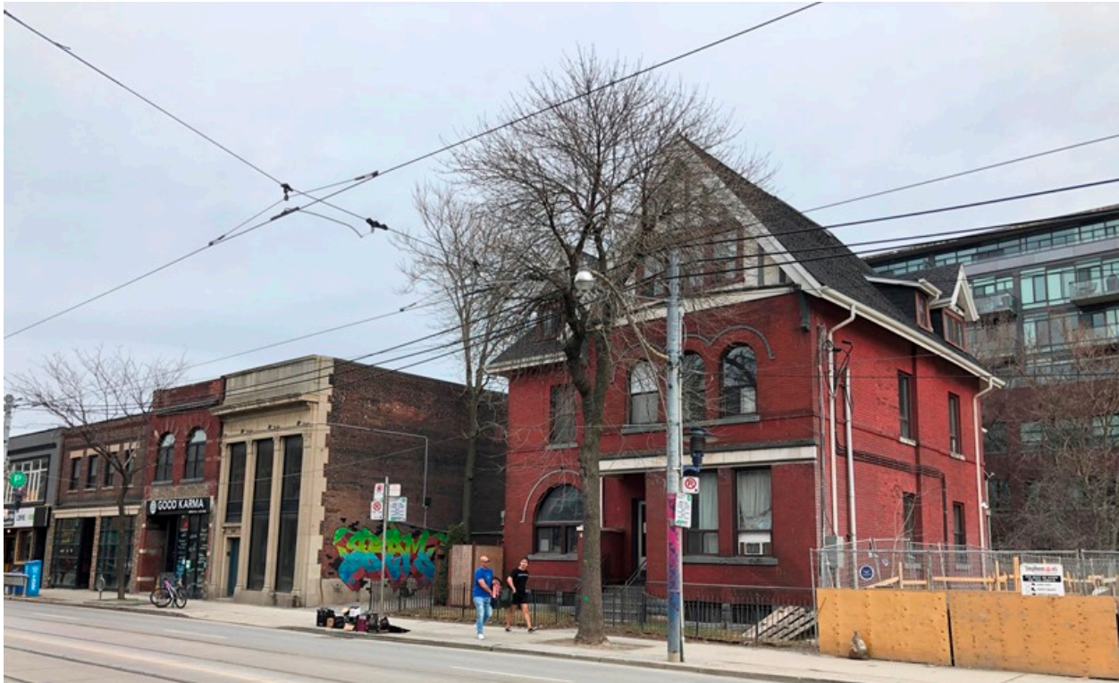
18. Context adjacent to the property at 685 Queen Street East: showing the historic 1920s bank and late 19th-early 20th century shop fronts to the east on the south side of Queen Street East (HP, 2021)
